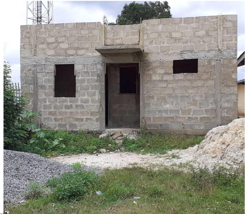
CONSTRUCTION OF 1NO-10-UNIT TOILET AT MOSEASO-ON-GOING
