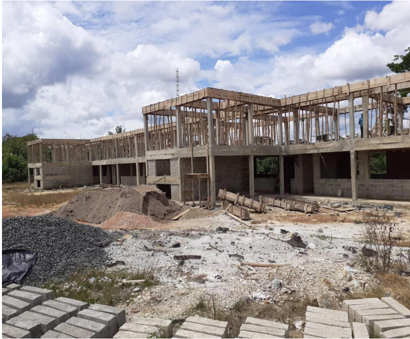
CONSTRUCTION OF 2 STOREY -12 UNIT CLASSROOM BLOCK AT ASECTECH
