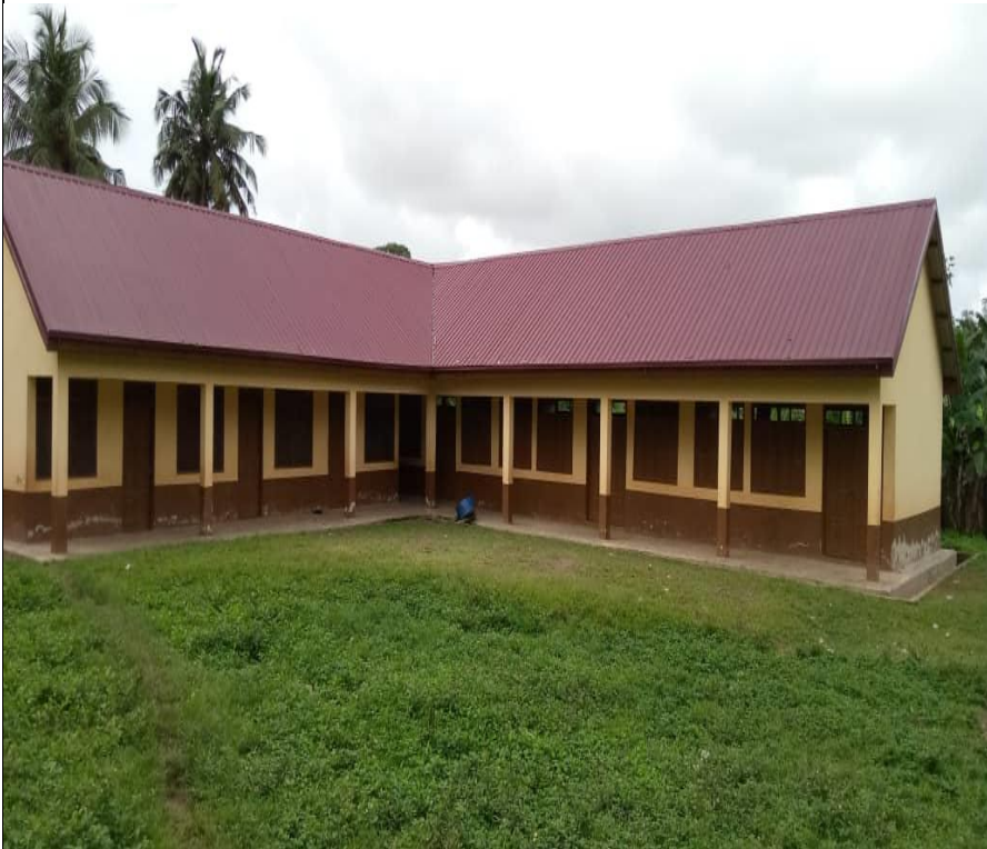
CONSTRUCTION OF 1 NO.3-UNIT CLASSROOM BLOCK WITH ANCILLIARIES FACILITIES AT KWABENG- COMPLETED
