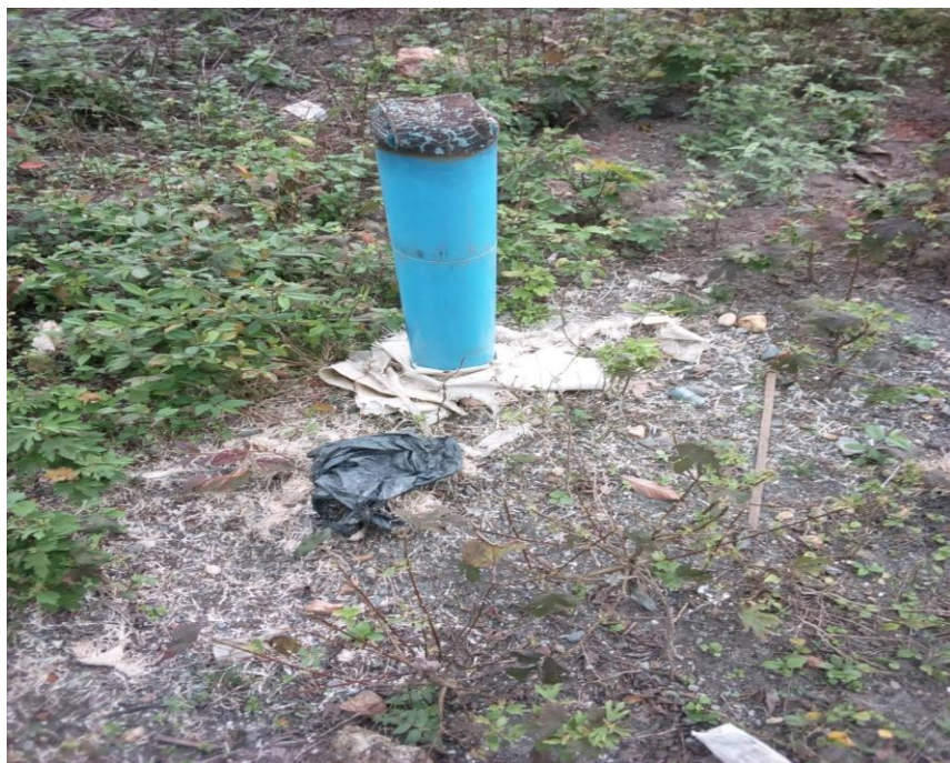
CONSTRUCTION OF MECHANIZED BOREHOLE AT TIGARIKROM-ON-GOING
