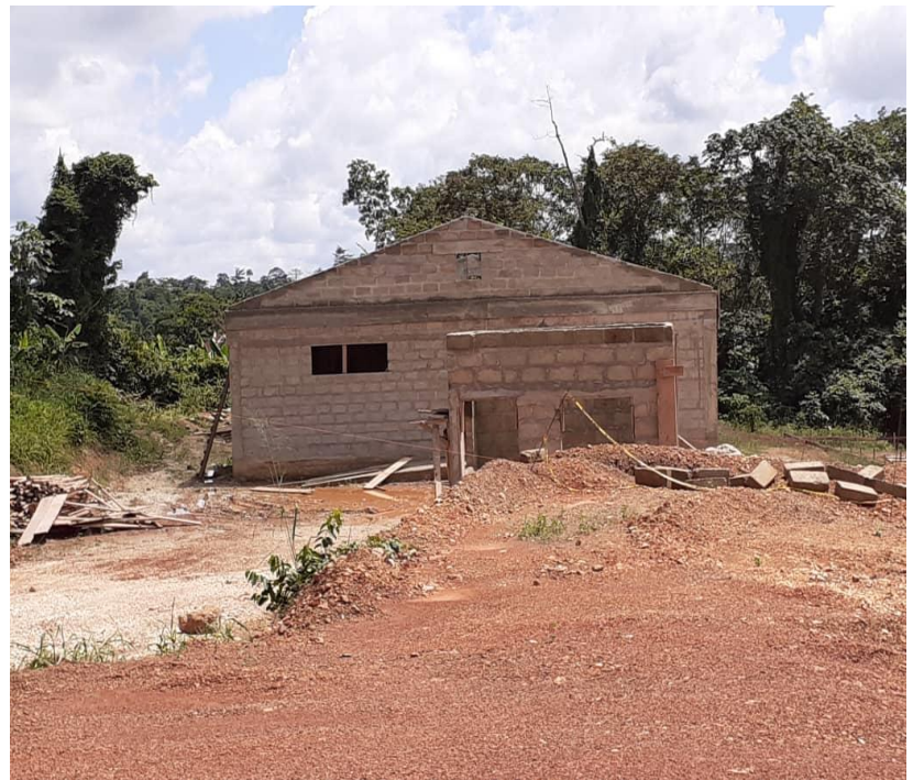
CONST. OF ELECTRICITY SUB-STATION @ ASANKRANGWA-ON-GOING
