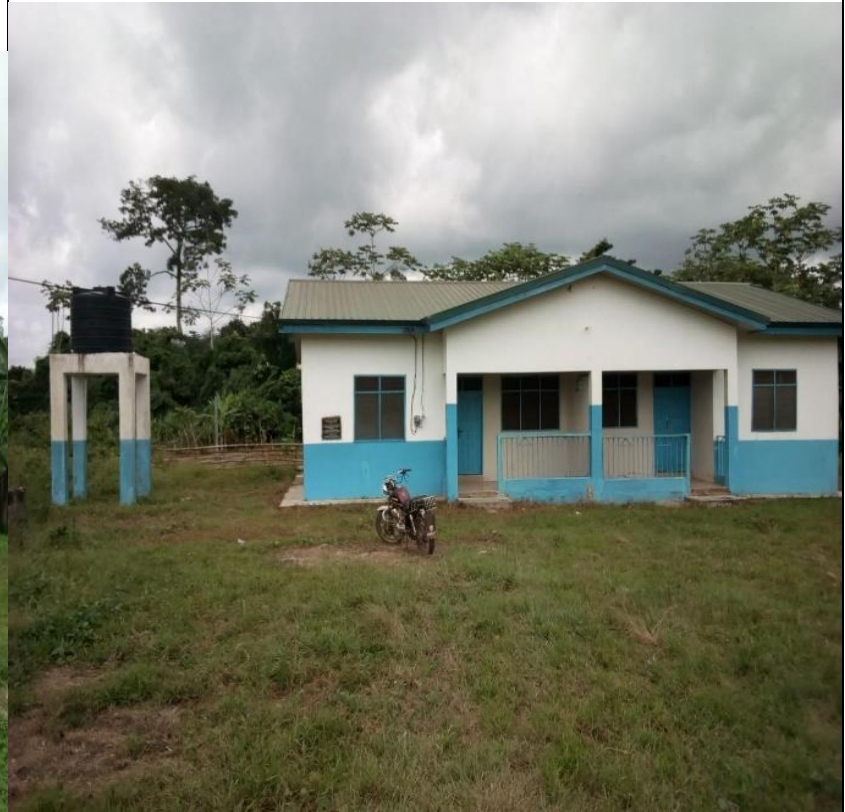
CONSTRUCTION OF TEACHERS QUARTERS WITH POTABLE WATER AT AMUAKU-COMPLETED
