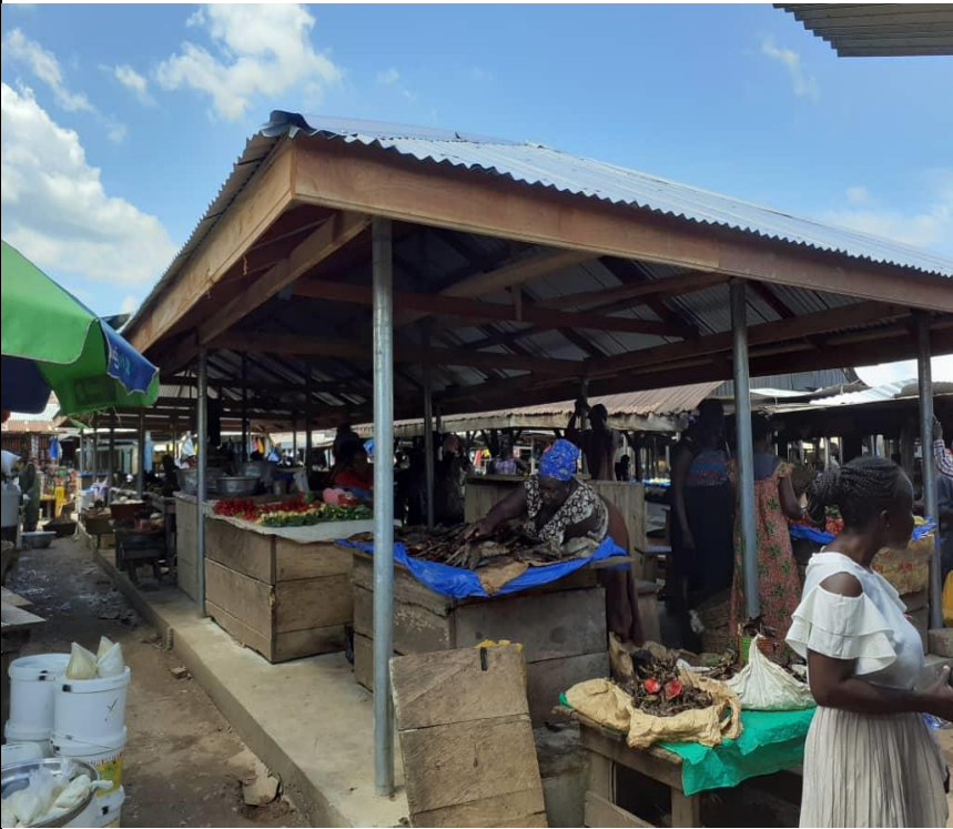
REFURBISHMENT OF MARKET SHED AT ASANKRANGWA MARKET CENTER-COMPLETED
