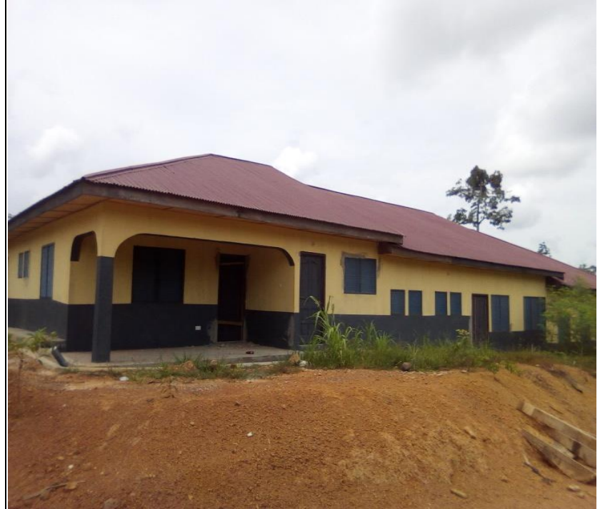
CONSTRUCTION OF 1NO. CHPS COMPOUND AT WOMEN-NO-GOOD- ON-GOING
