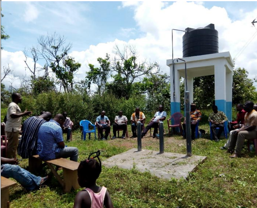
1 NO. MECHANIZED BOREHOLE AT NKEKENSU- COMPLETED
