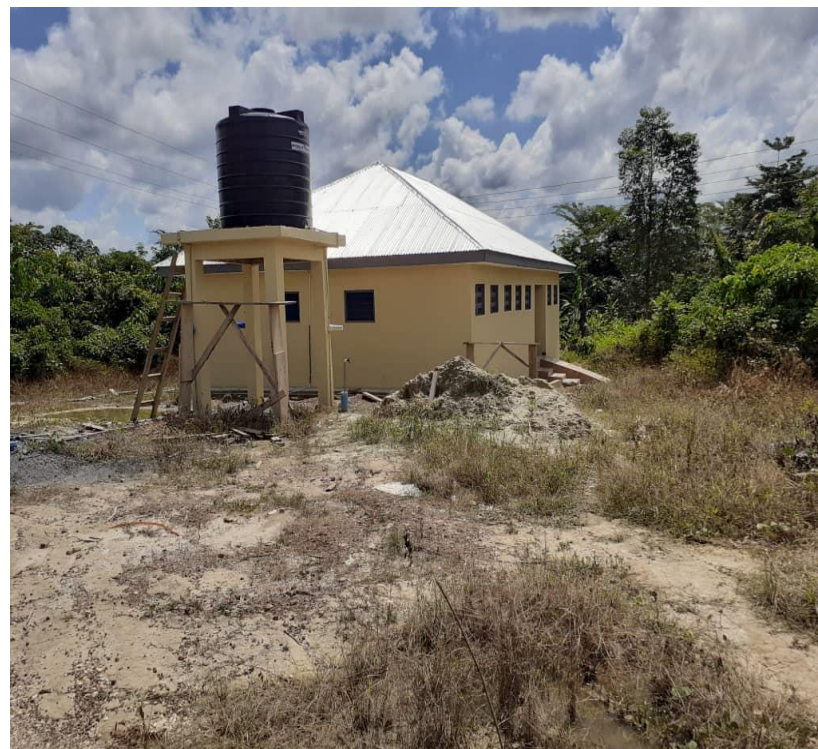
CONST. OF 1 NO. LAVATORY LIGHT INDUSTRIAL AREA, ASANKRANGWA- COMPLETED
