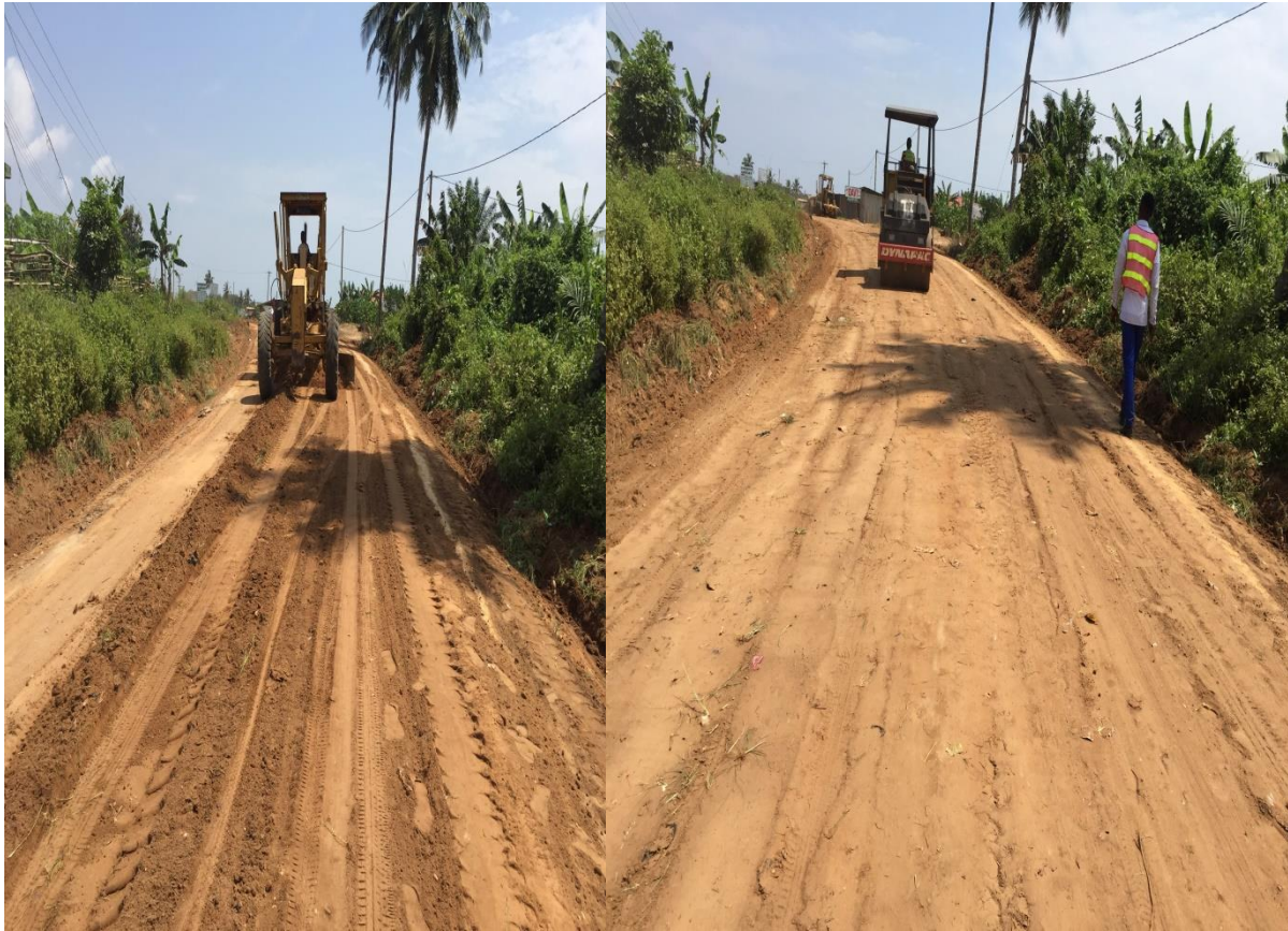
Grading Works on Selected Roads in EKMA
