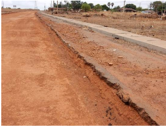
After Removal of Cement stabilized Base Course on Bafilo Bypass in Togo
