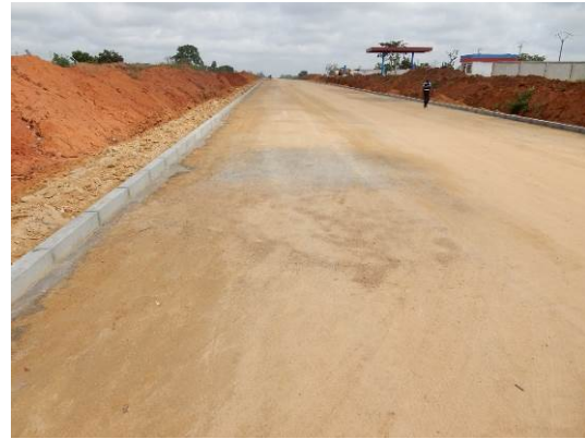
Completion of Cement Stabilized Sub-base Course on Lomé - Tsevie Section in Togo
