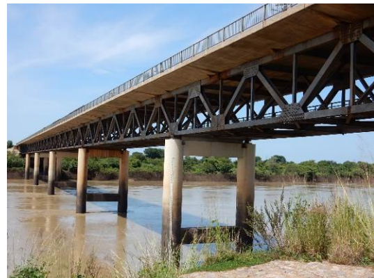
Yapei Bridge in Ghana
