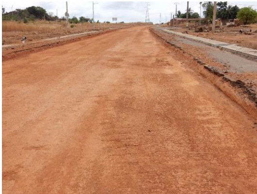
Bafilo Bypass in Togo
