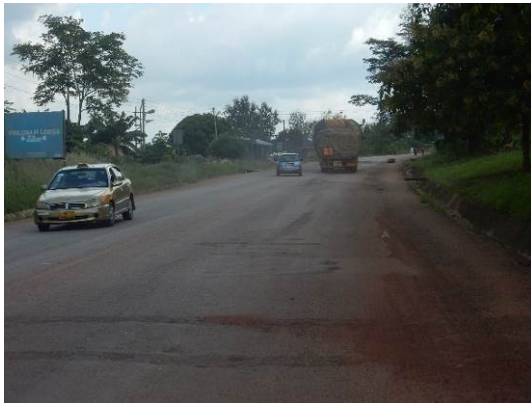
DBST on Western Corridor in Ghana
