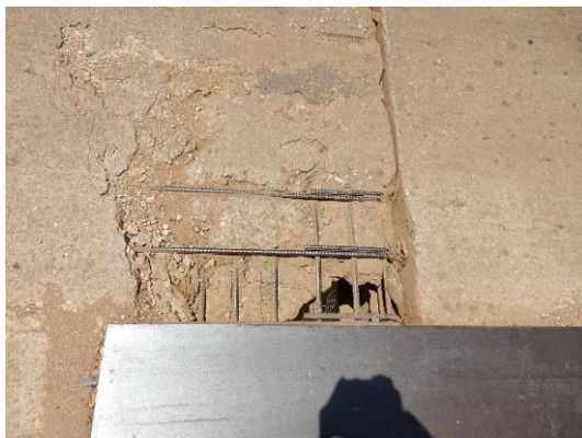
Buipe Bridge in Ghana
