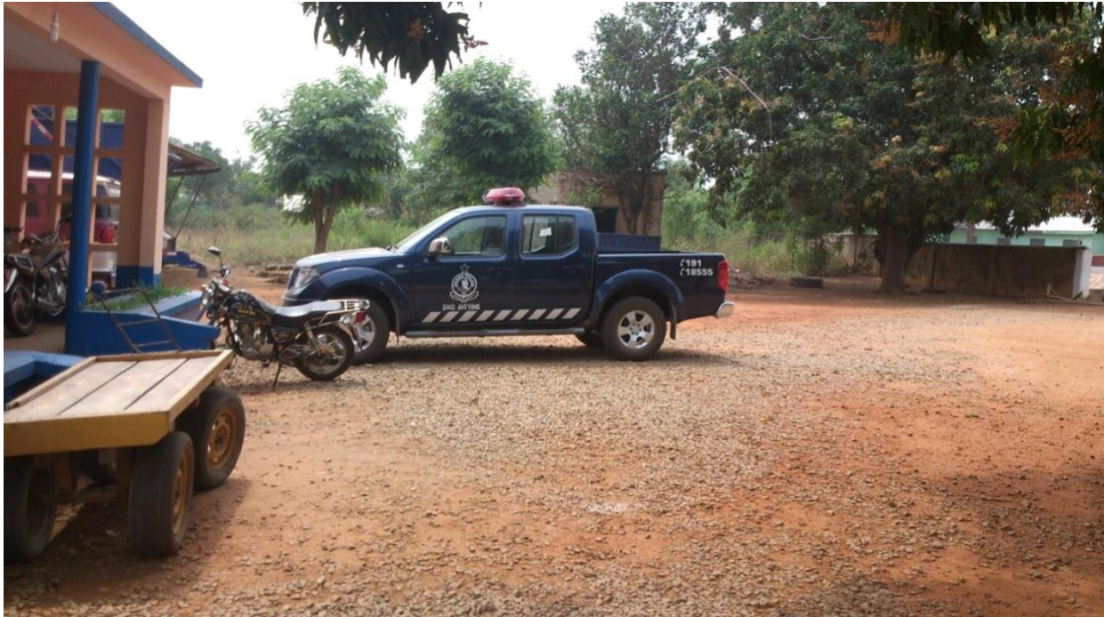
Figure 1.25 District Police Headquarters, Aveyime
