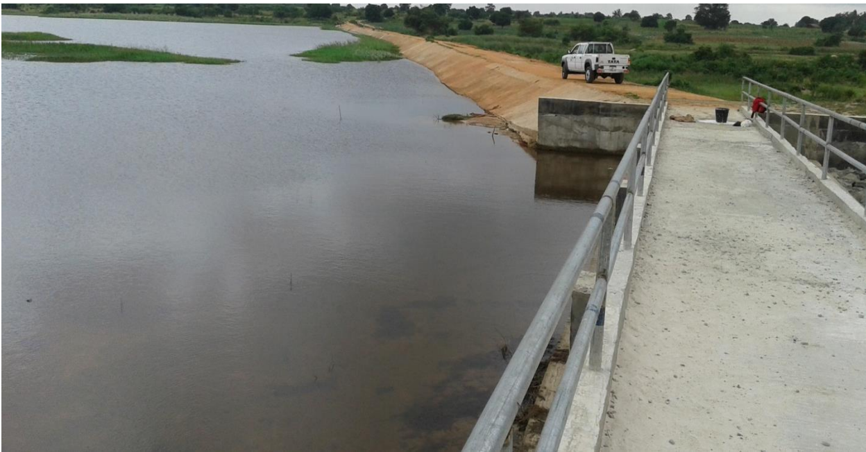
PICTURE OF THE OHAWU DAM WITH SPILL OVER WALKWAY
