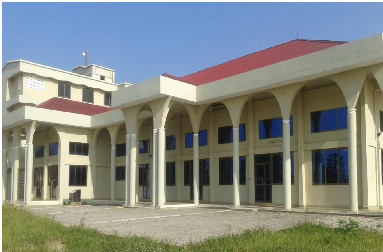
THE MUNICIPAL ASSEMBLY AND HALL COMPLEX AT DZODZE-KAVE
