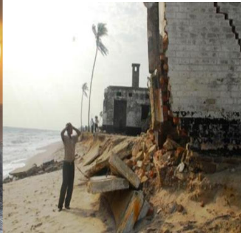
Destructions cause by tidal wave
