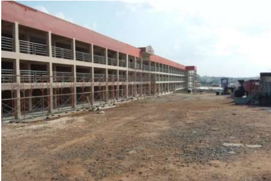
Figure 8: Ho Central Market under construction
