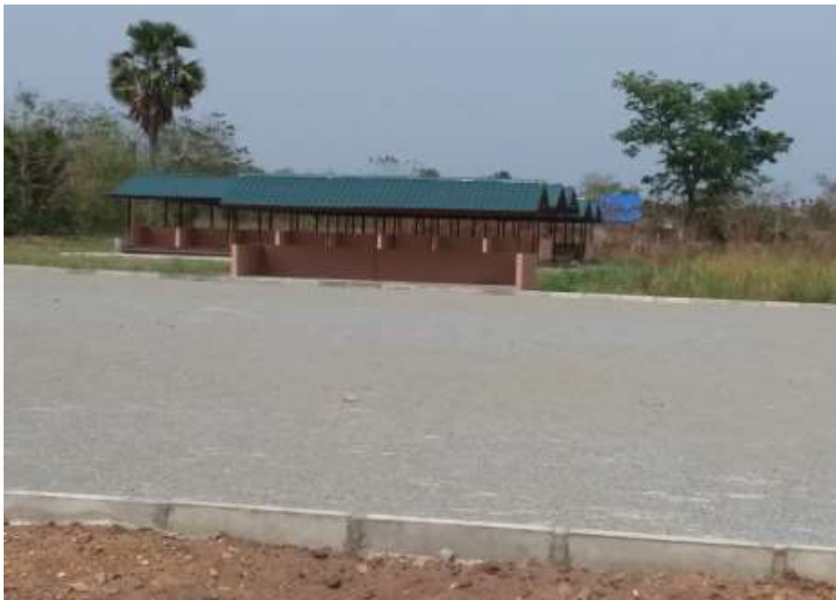
Figure 9: Newly completed markets stalls with taxi rank - Sokode Gbogame
