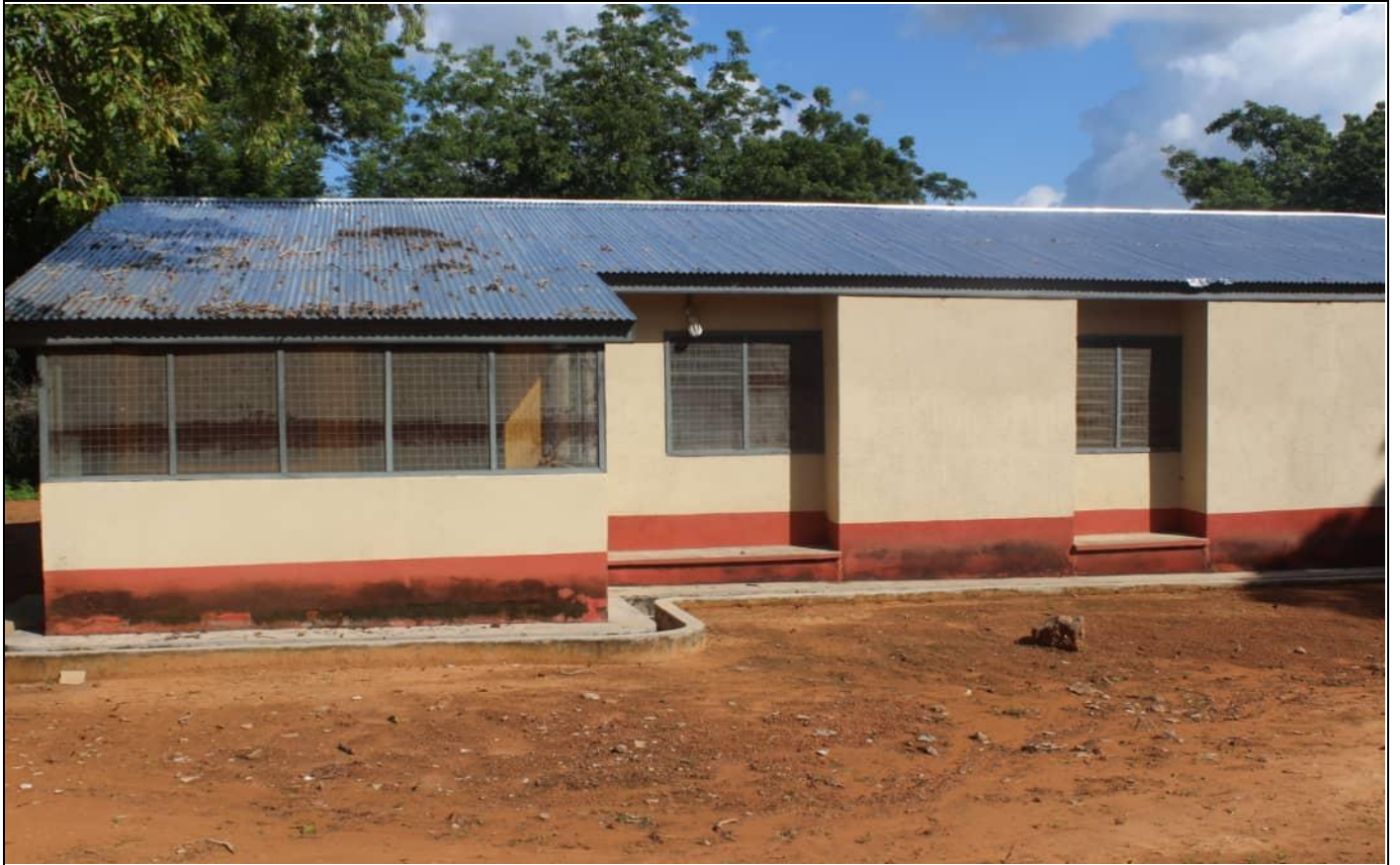
REHABILITATION OF HEALTH DIRECTOR'S BUNGALOW (FUNDED WITH DACF)
