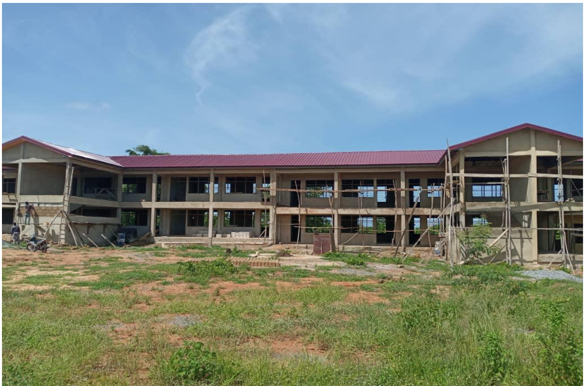
12-UNIT CLASSROOM EMERGENCY BLOCK @ DAMONGO SHS (GETFUND
