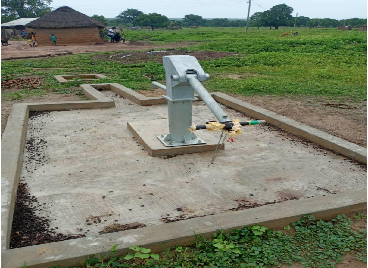
BOREHOLE @ JONOKPONTO (FUNDED BY WORLD VISION)
