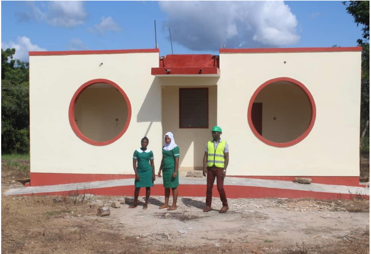
10 SEATER WC TOILET WITH SOLAR POWERED BOREHOLE & S LIGHTENING @ DAMONGO NURSES COLLEGE (IPEP)
