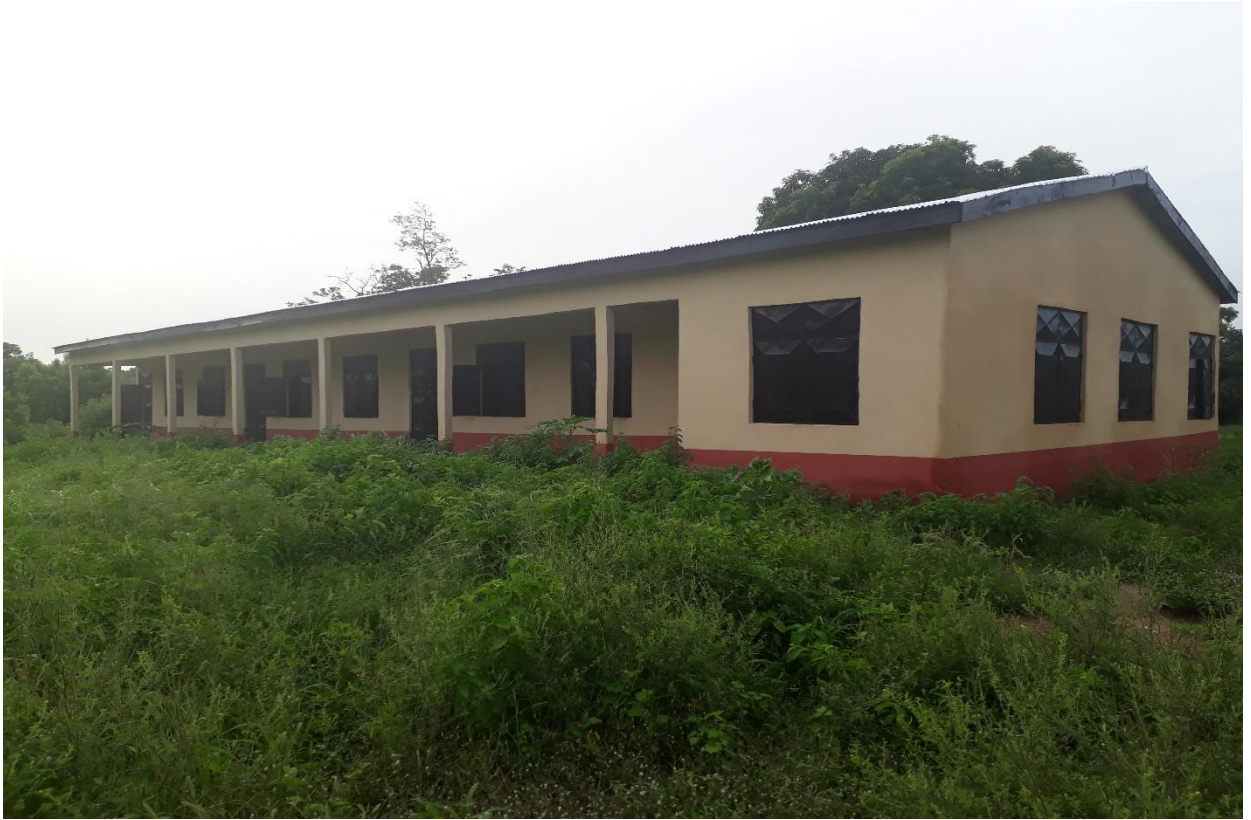
3-UNIT CLASSROOM BLOCK WITH ANCILLARIES @ DAMONGO MODEL SCHOOL - ABINGAKURA
