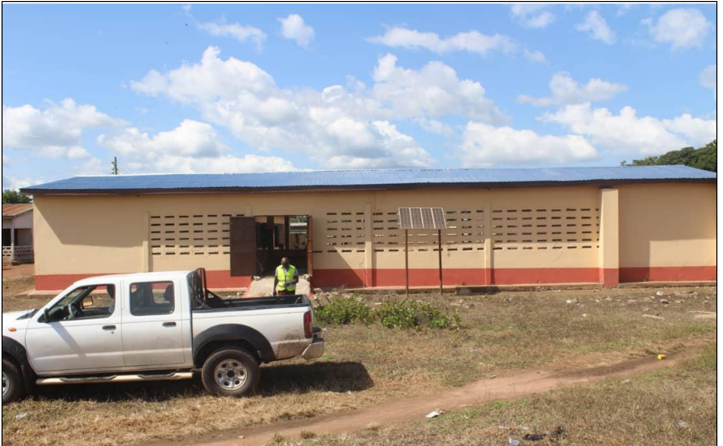
REHABILITATION OF HEALTH CENTER @ BUSUNU (FUNDED WITH DACF)
