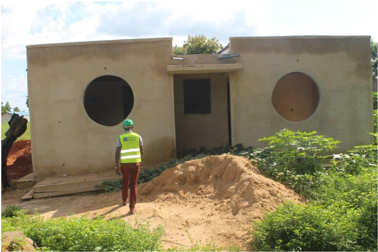
10 SEATER WC TOILET WITH SOLAR POWERED BOREHOLE & LIGHTENING @ NDESCO (IPEP)
