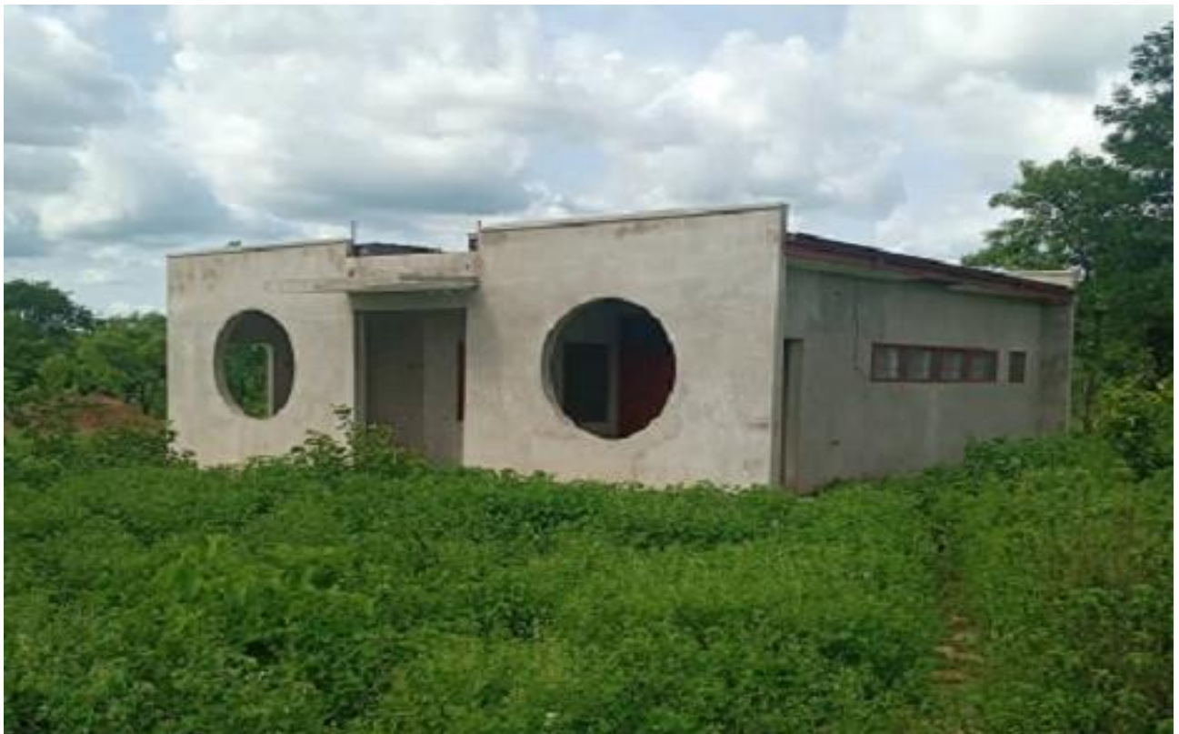
10 SEATER WC TOILET WITH SOLAR POWERED BOREHOLE & LIGHTENING @ LARIBANGA (IPEP)
