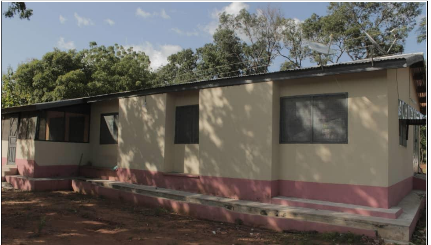
RENOVATION OF 1NO POLICE COMMANDER'S BUNGALOW @ DAMONGO (FUNDED WITH DACF)
