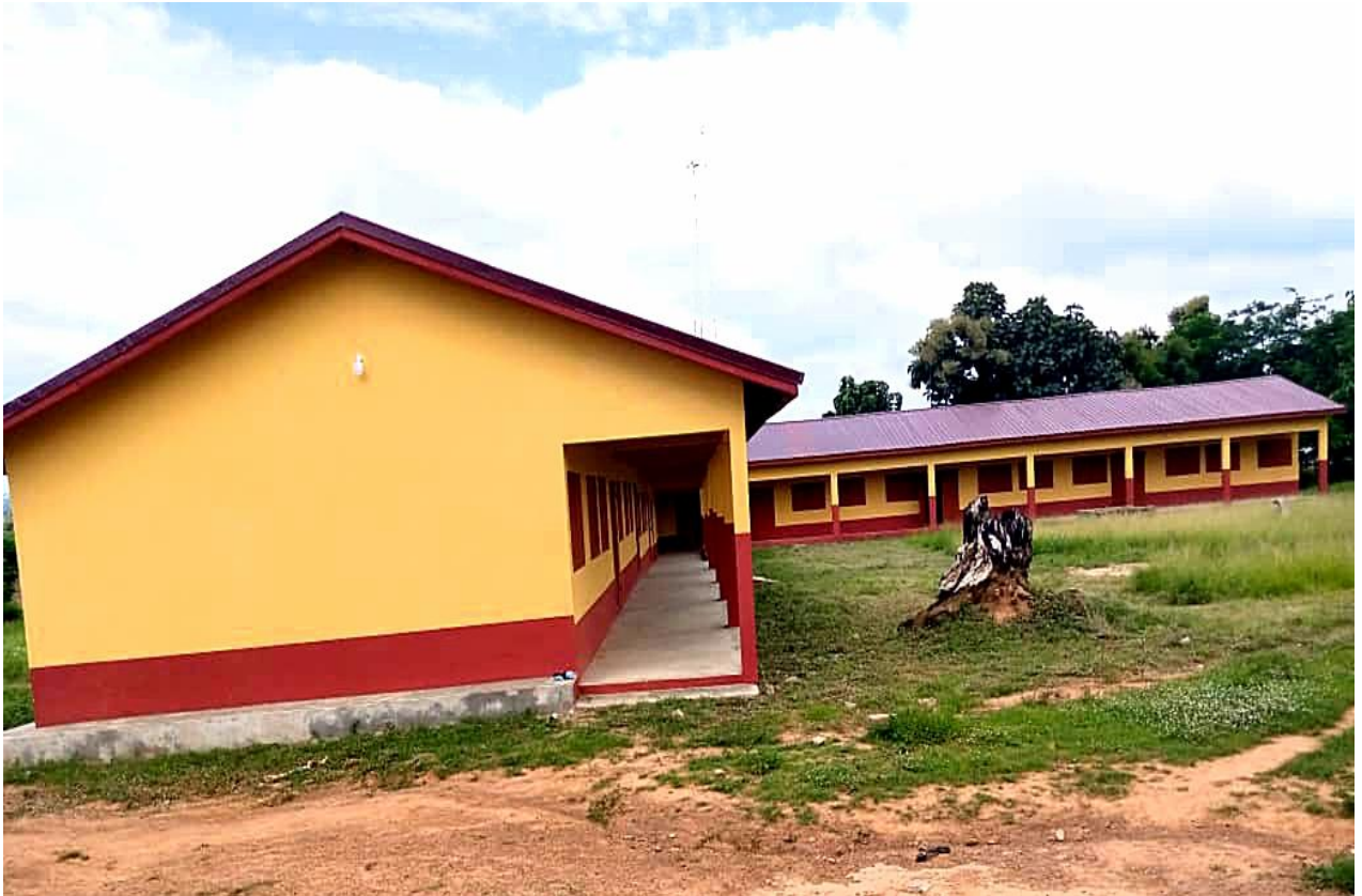
CONSTRUCTION OF 1 NO 6 UNIT CLASSROOMS BLOCK AT ABOTOASE
