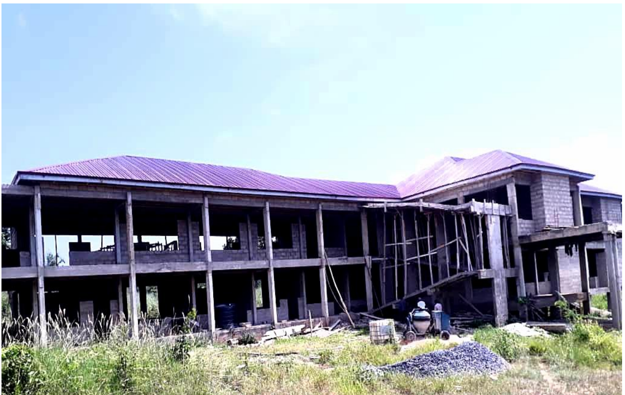
CONSTRUCTION OF ASSEMBLY OFFICE COMPLEX AND HALL AT NKONYA
