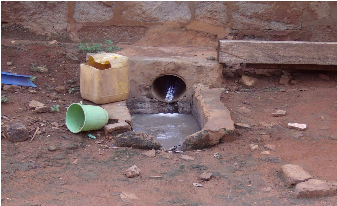
Picture 1: Shows a typical Bathroom sullage collection point in use (Courtesy of MPCU, NSMA)
