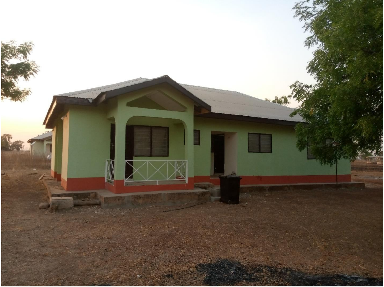
STAFF BUNGALOW RENOVATED
