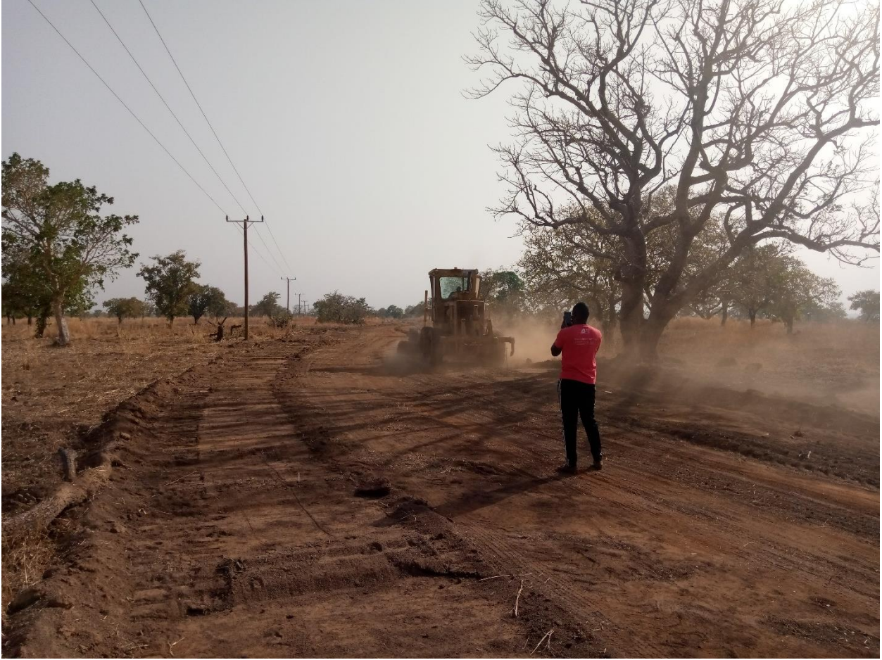
RESHAPING OF NYANGBOLO -TULINGA – SHEBO FEDER ROAD
