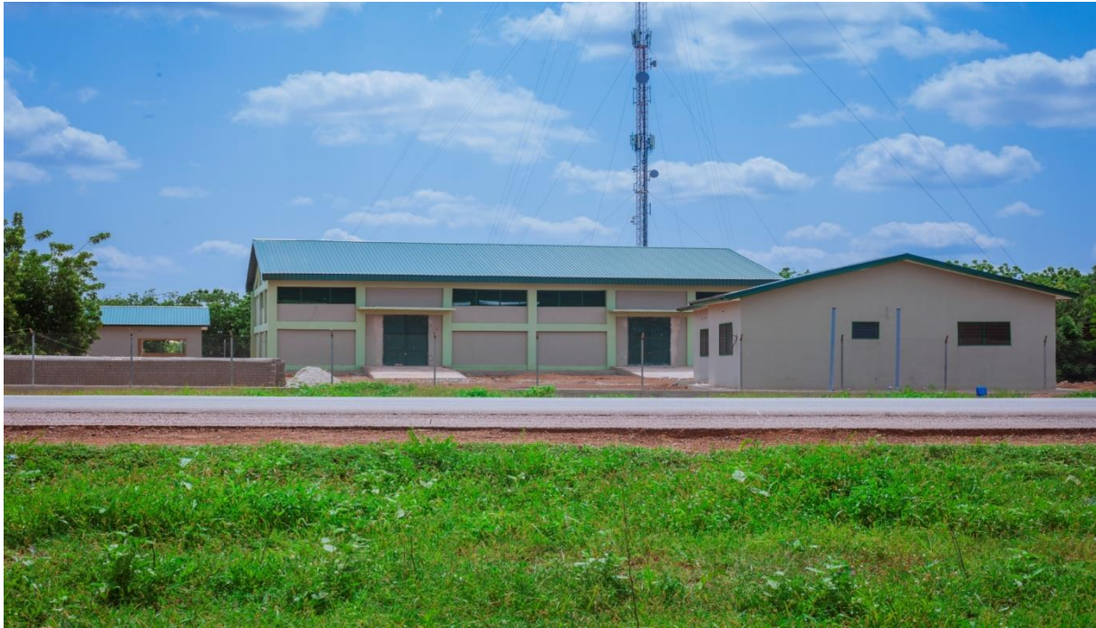
Completed warehouse at Walewale
