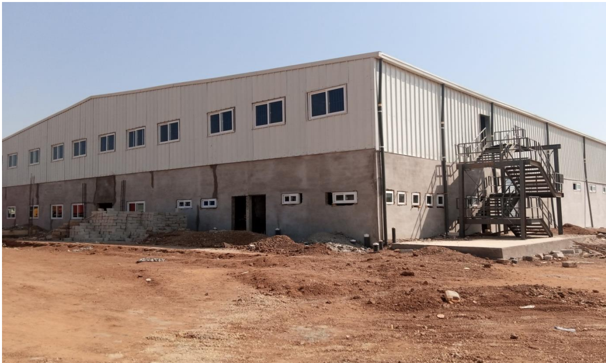
On-going construction of watermelon processing factory
