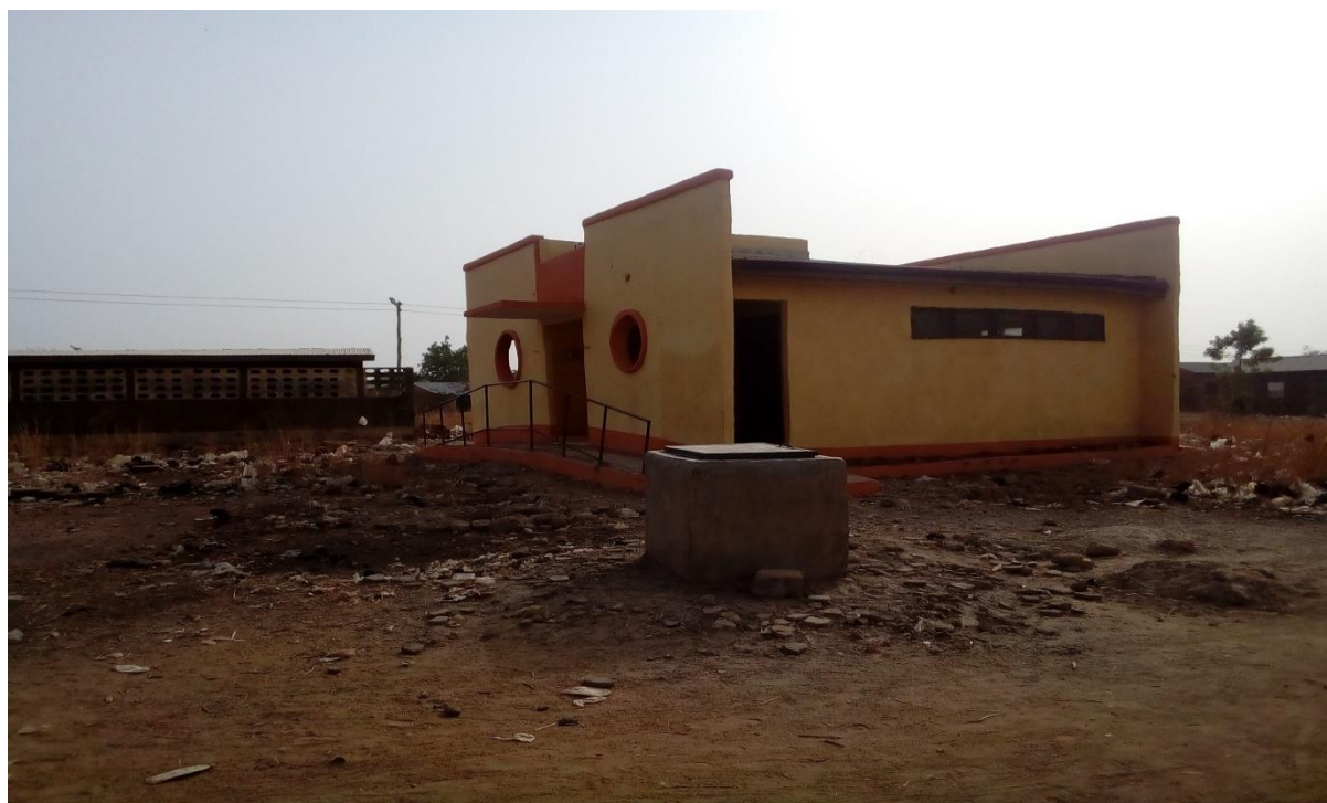
Figure 2.11: On-going construction of WC toilet at Chereponi new market
