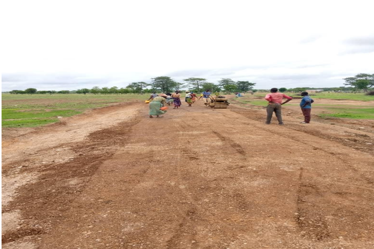
Figure 2.7: Rehabilitation of Sangbana junction-Sangbana Feeder Road (2km)
