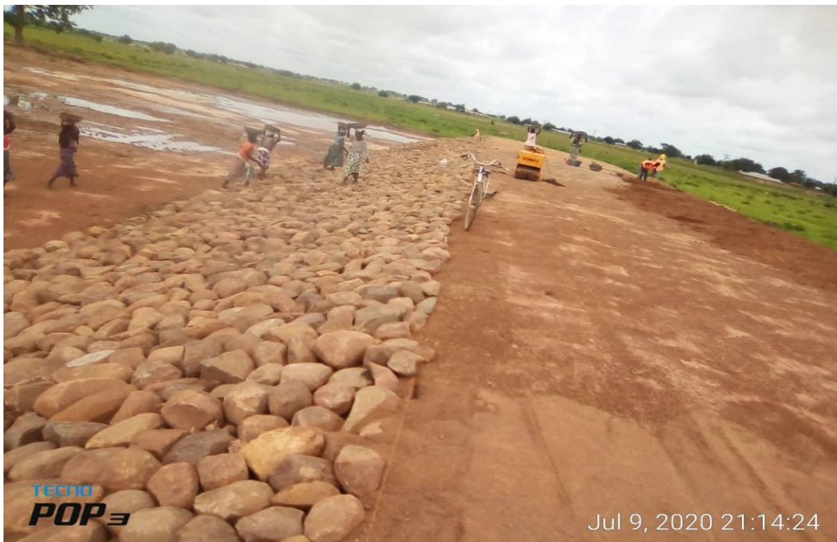
Figure 2.6: On-going Rehabilitation of Small Earth Dam at Wenchiki
