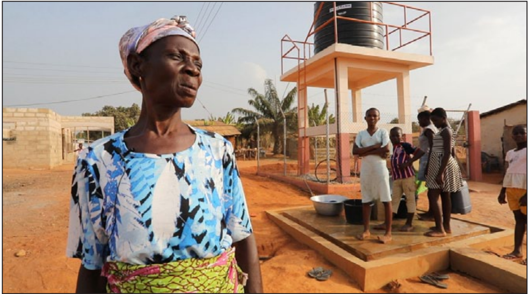
Akua Osaa, water vendor at Gambia no 1, Asutifi North. Sales at community taps raise money to cover minor repairs and maintenance.
