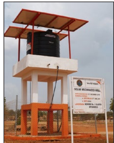
Solar powered mechanised borehole in Kenyasi No. 2
