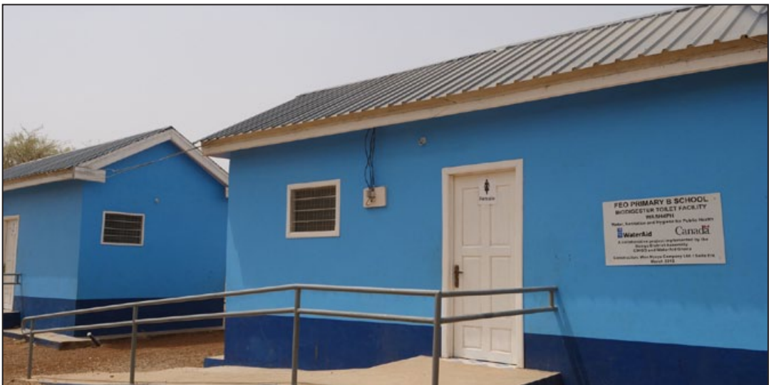
Modern flush toilets with menstrual hygiene facilities at Foe Primary School B, in Bongo District
