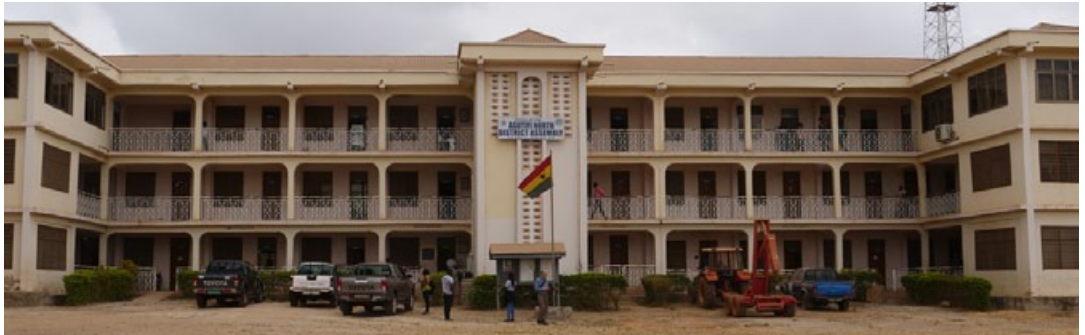
Asutifi North District Assembly, home of the ANAM initiative to achieve SDG 6.
