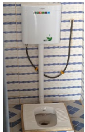
Flush toilets at Foe CHPS
