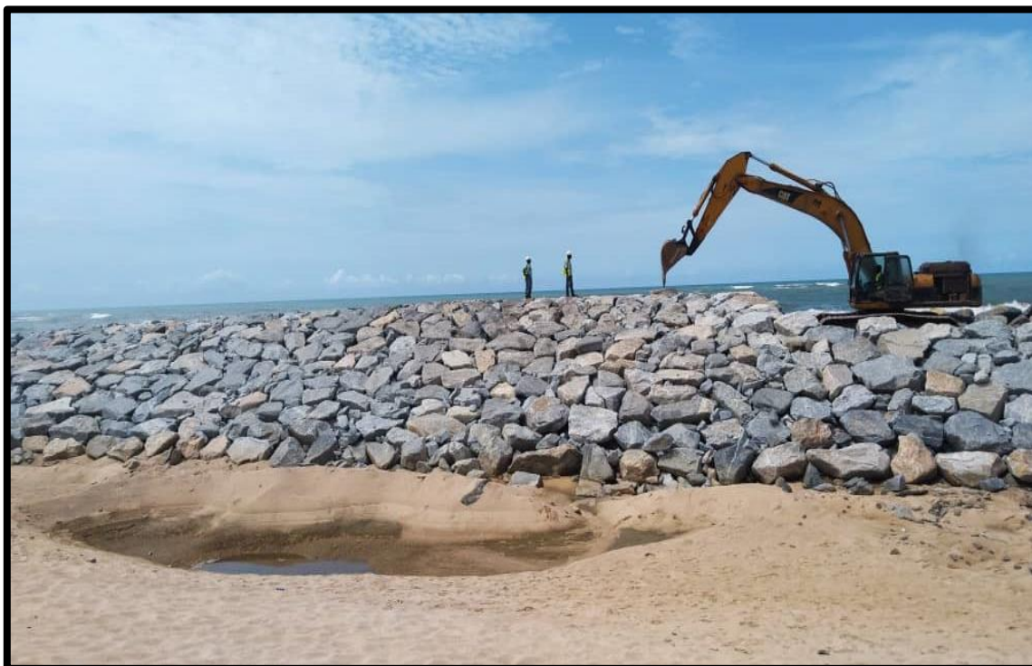
Figure 5: A Section of the completed Revetment at Amanful Kumah
