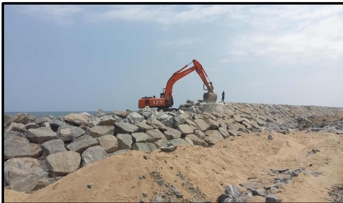
Figure 6: A Section of the ongoing works at Cape Coast
