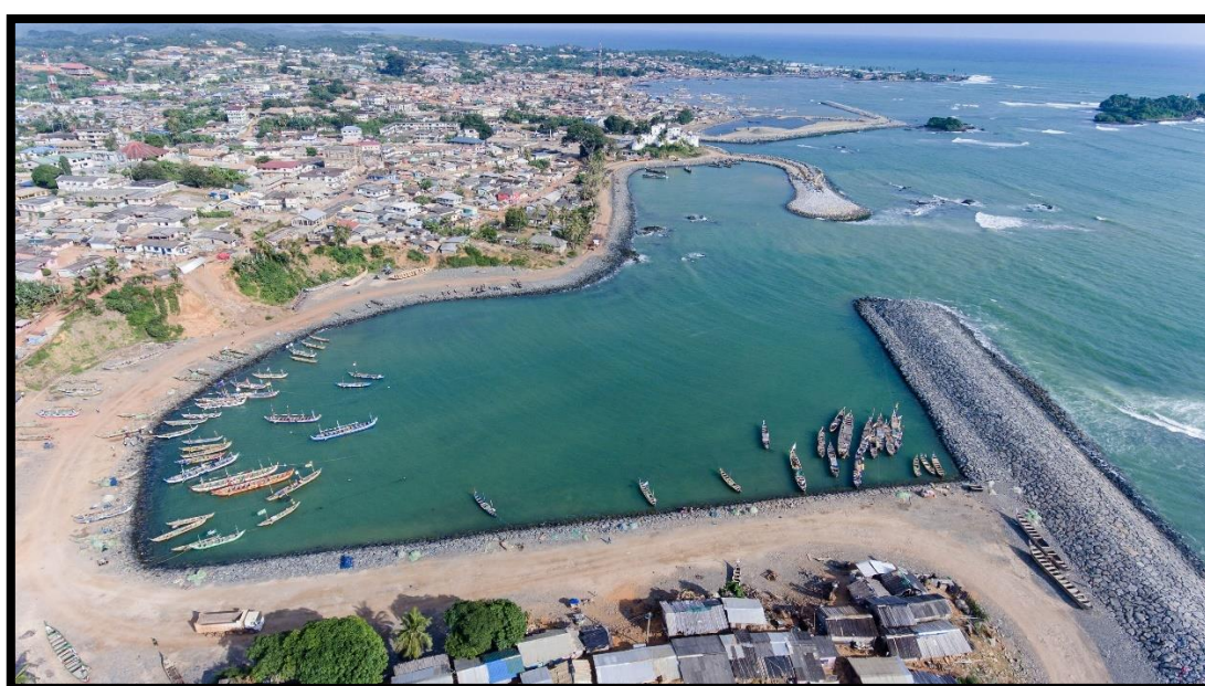
Figure 3: Axim Coastal Protection Project
