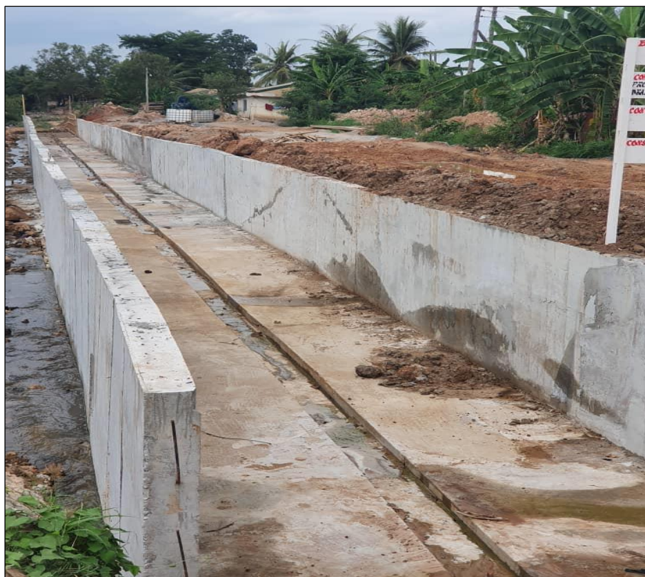
Figure 2: On-going Construction Work on Kordjor Drainage Channel
