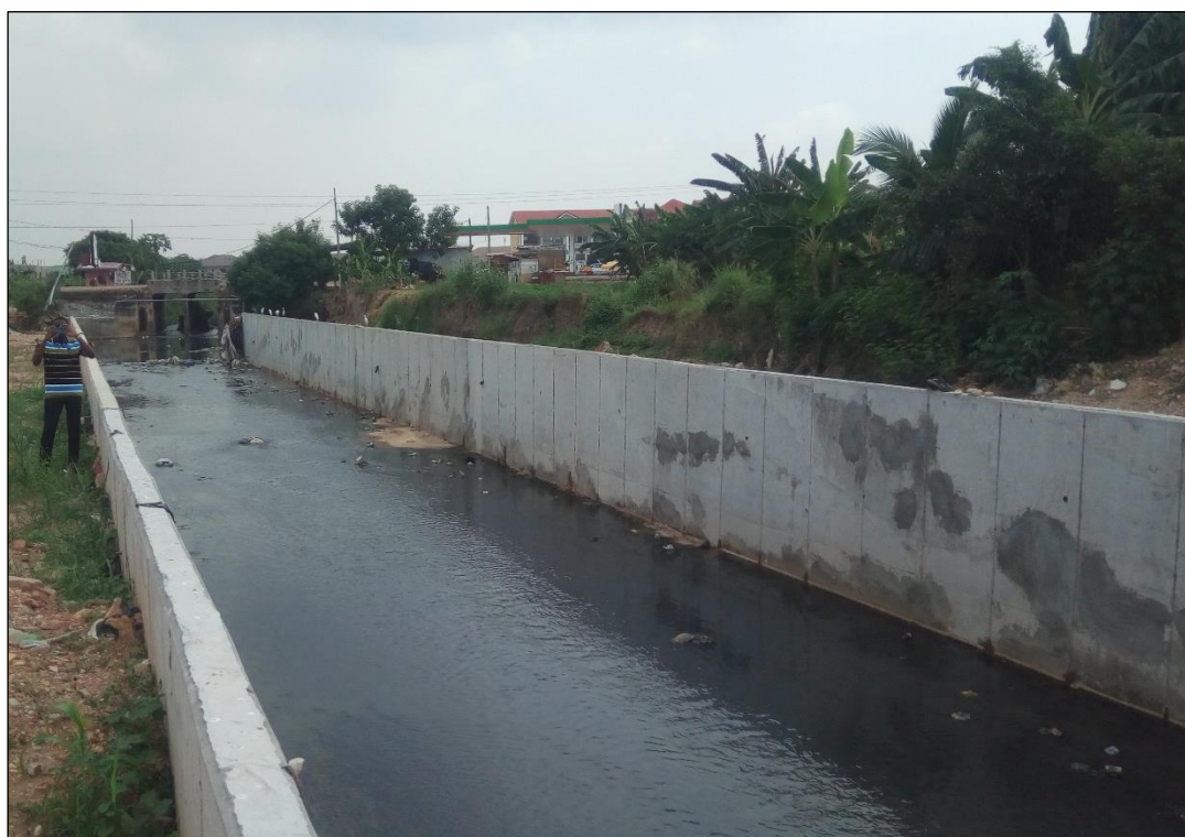
Figure 1: Completed Storm Water Drainage Channel
