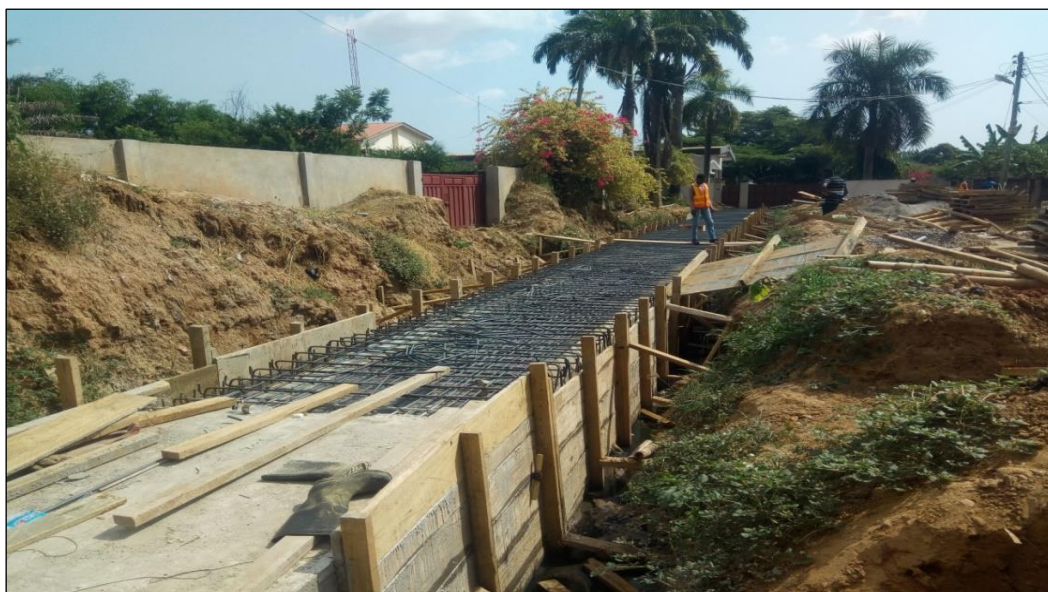
Figure 2: On-going Construction Work on Kordjor Drainage Channel
