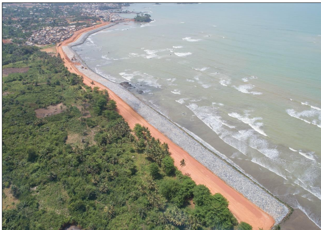
Figure 6: A Section of the Completed Revetment Wall with Lateritic Backfilling at Axim
