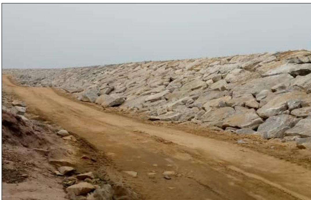
Figure 3: New Takoradi (Elmina) Coastal Protection Project (Phase II)
