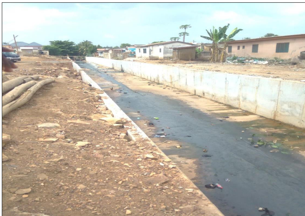
Figure 1: Completed Storm Water Drainage Channel
