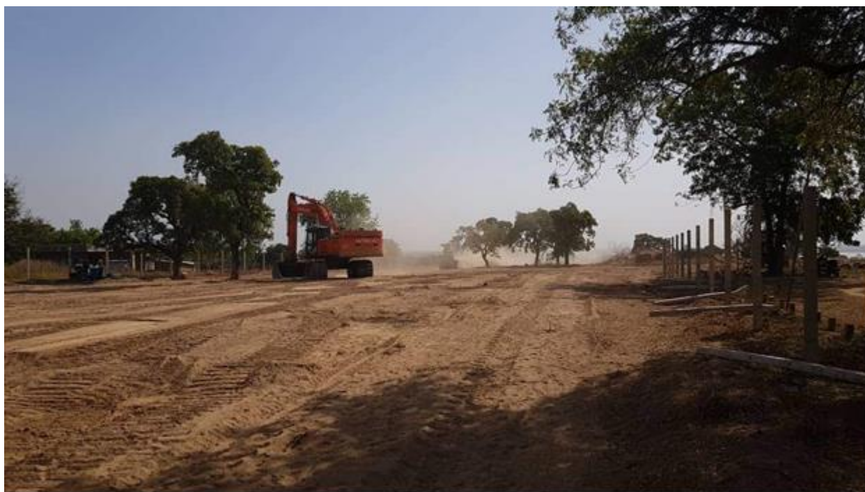
1. Clearing of Site for the construction of WTP @ Tono
