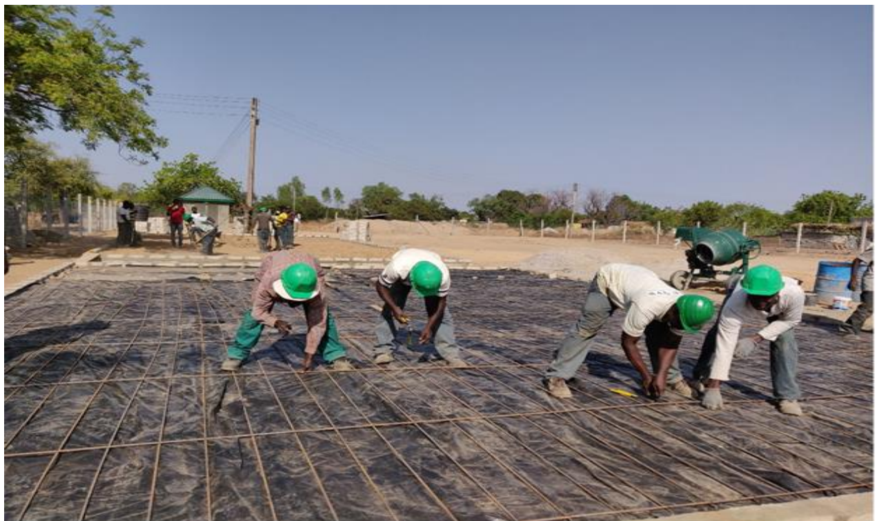
1. Preparation of a Mat Foundation for the Contractor's office
