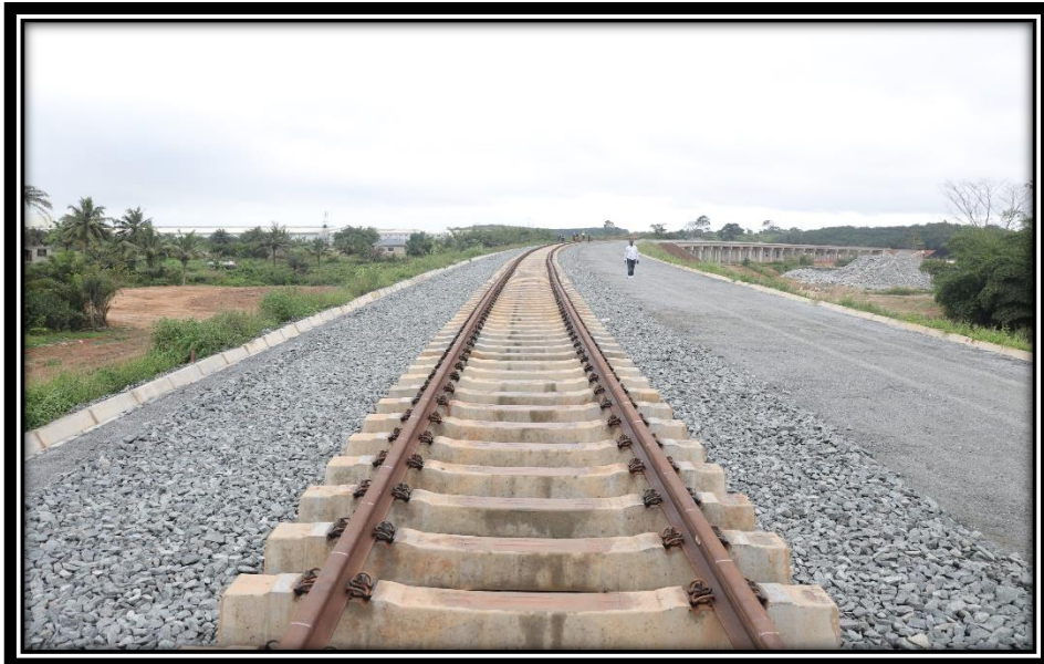
Track works at Eshiem on the Western Railway Line
