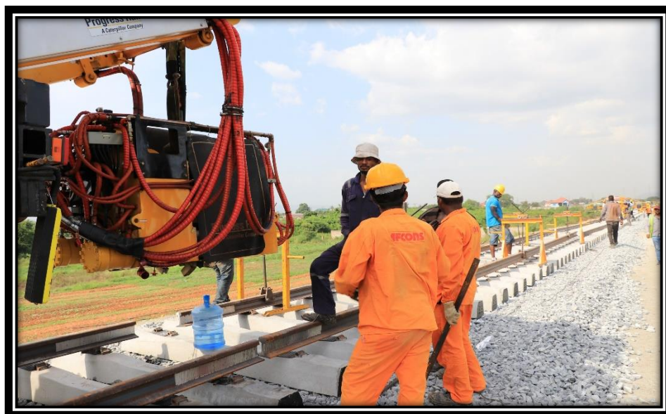
Track Laying Works on the Tema-Mpakadan Railway Line
