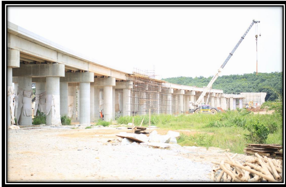
Eshiem Viaduct (Railway Bridge)
