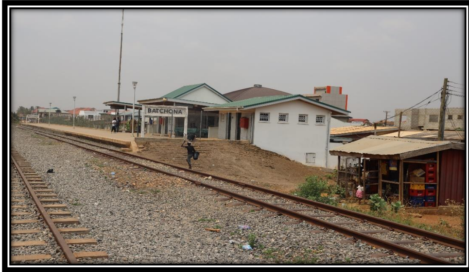
Rehabilitated Accra-Tema Line (Batchona Railway Station)
