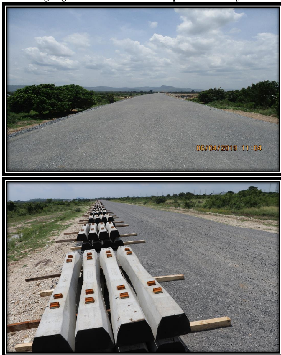
On-going construction of Tema – Mpakadan railway line
