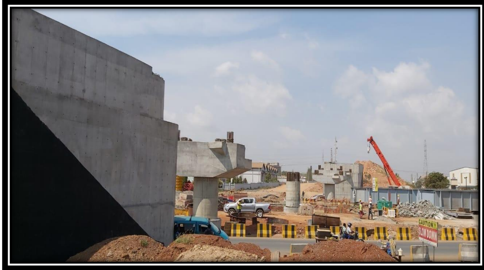
Construction of Railway Bridge across near Tema Motorway Round About
