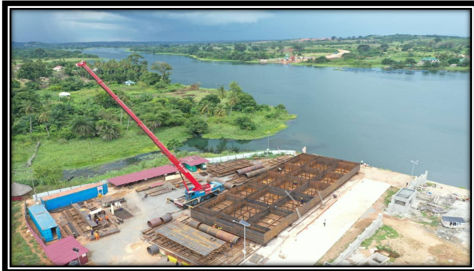
Construction of Railway Bridge across Volta River
