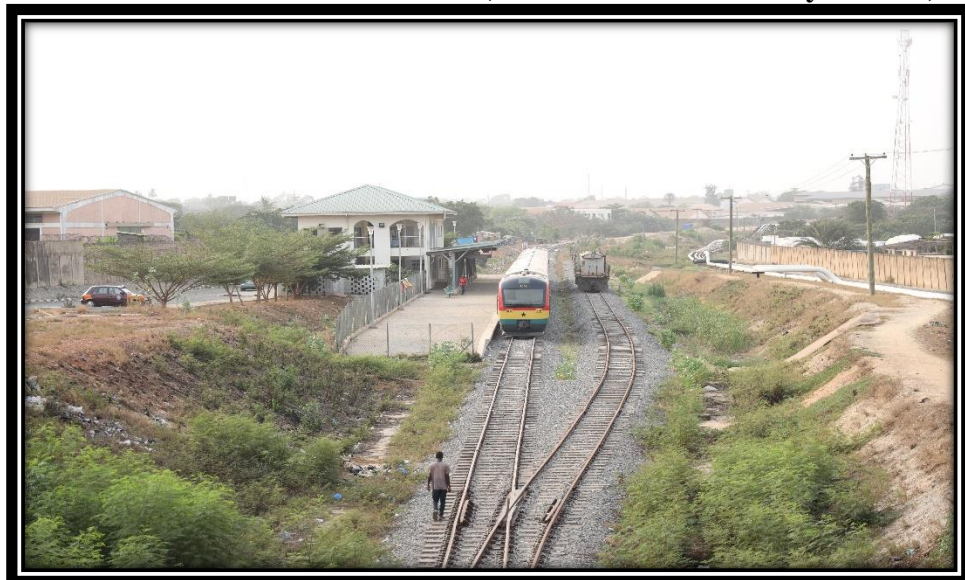
Rehabilitated Accra-Tema Line (Tema Comm. 1 Railway Station)
