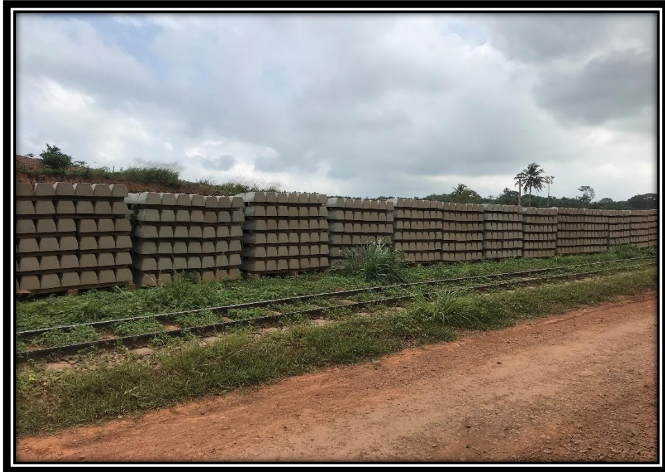
Stock-pile of concrete sleepers on site ready to be laid
