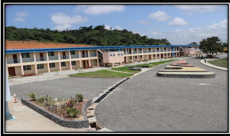
Rehabilitated Classroom Block
