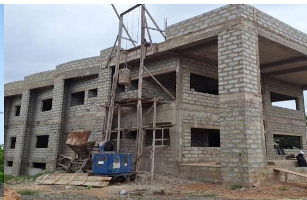
Construction of Tema District Office
