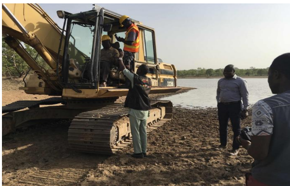
Hon Minister breaking ground for construction of dam, Kakiase
