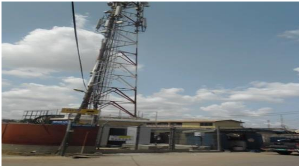
Monitoring of Telecommunication Masts
