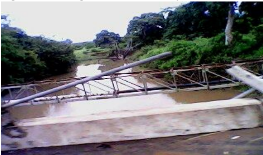
Figure 8: Showing a section of River Ayensu in the district
