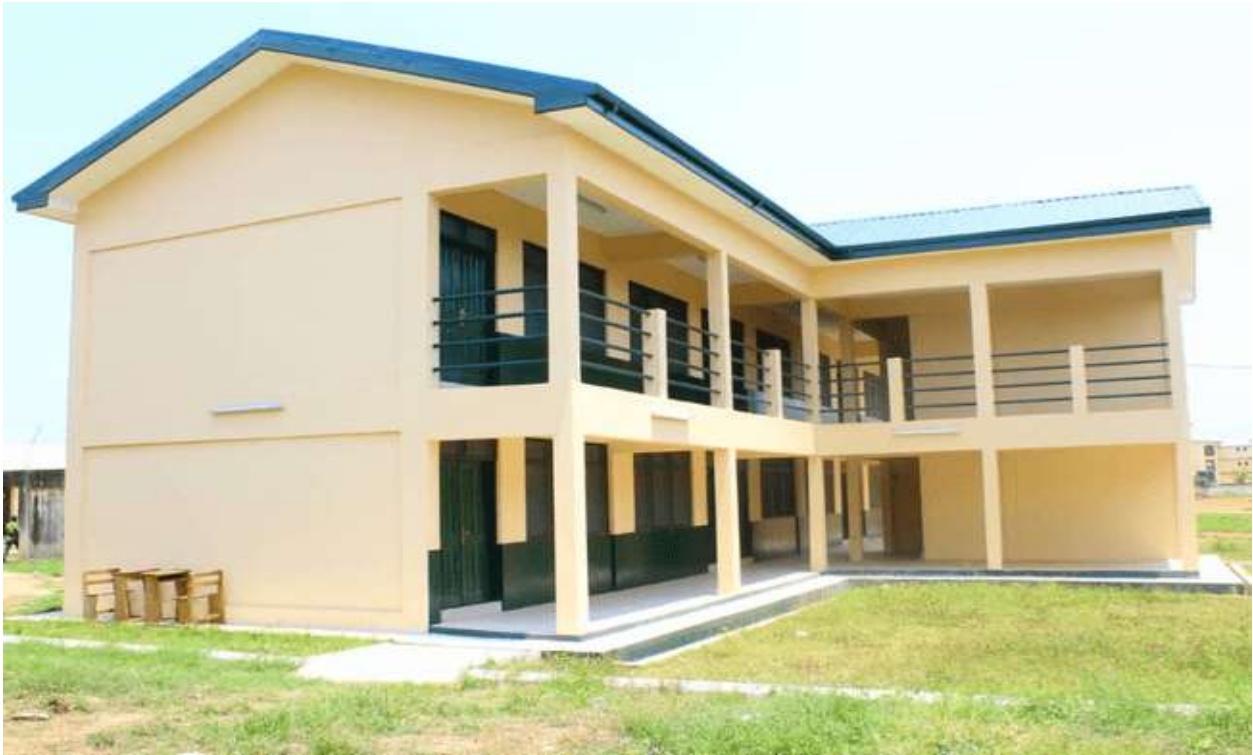
Construction Of 2-Storey 6-Unit Classroom Block at Tema Senior High School (Comm. 2)
