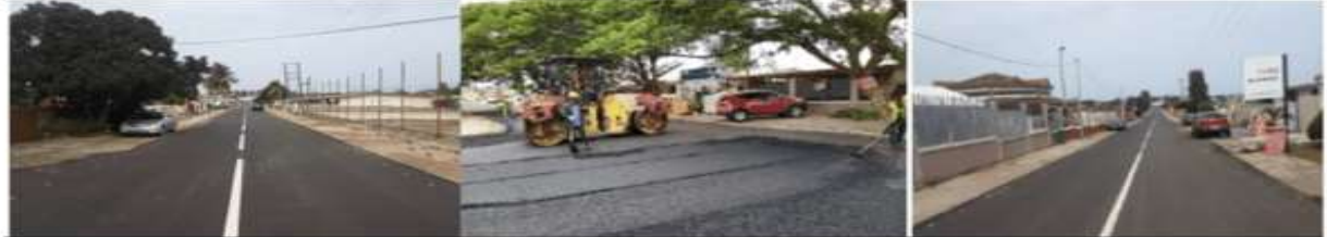
Asphalt works at Friday's Pub area
