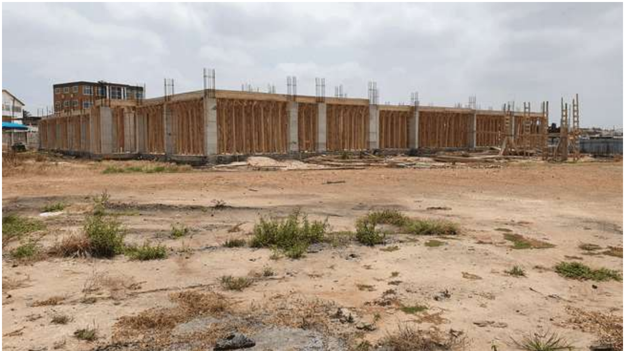
Construction of 3-Storey Office Administration Block for TWMA
