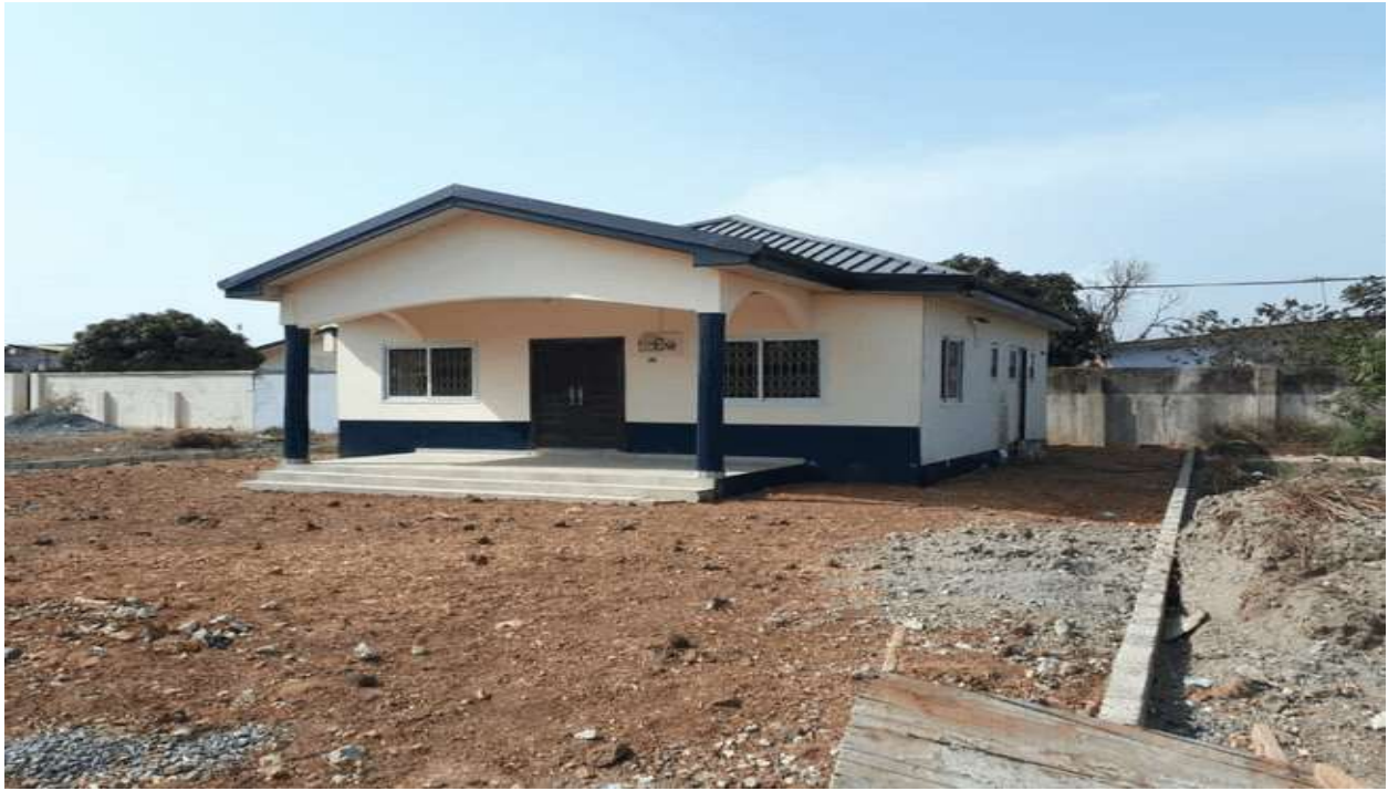
Construction of Police Station at Community 14 (Regimanuel) Sakumono
