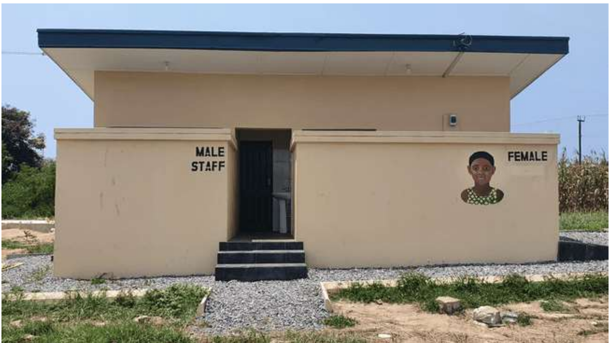
Construction of 10-Seater WC Toilet Facility at Tema Senior High School Comm. 2
