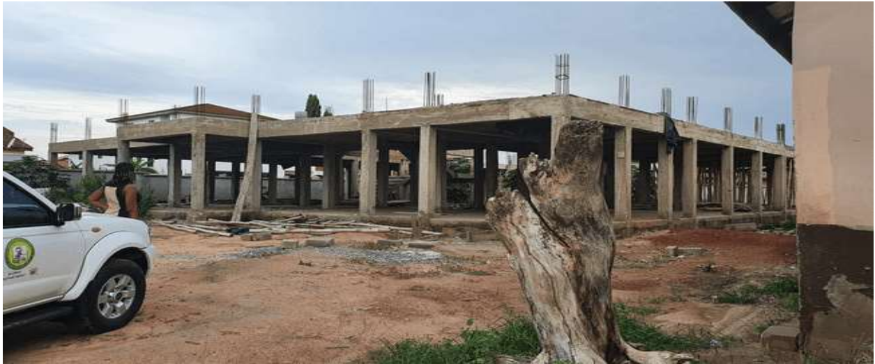
Construction Of 2-Storey 12-Unit Classroom Block at Lashibi Basic School Complex
