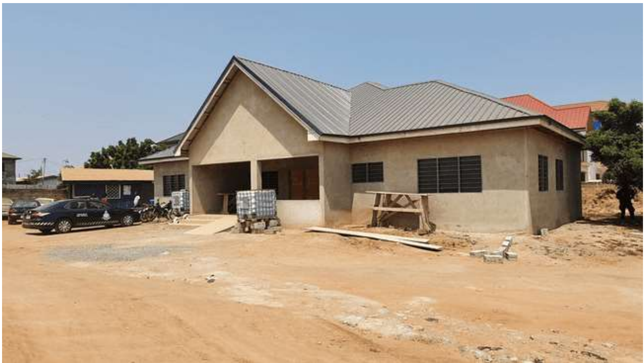
Construction of Police Station at Kanewu – Adjei Kojo
