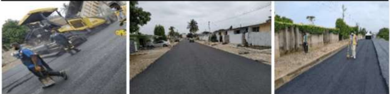
Asphalt works at Sakumono 3 rd Chapel Square Link
