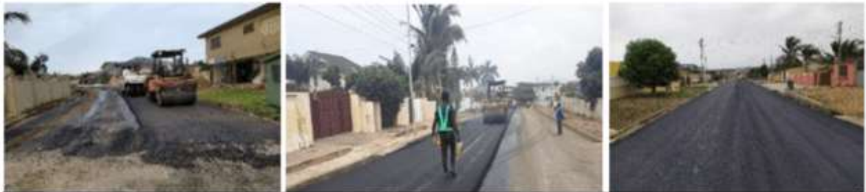
Asphalt works at Sakumono 4 th Chapel Square Link
