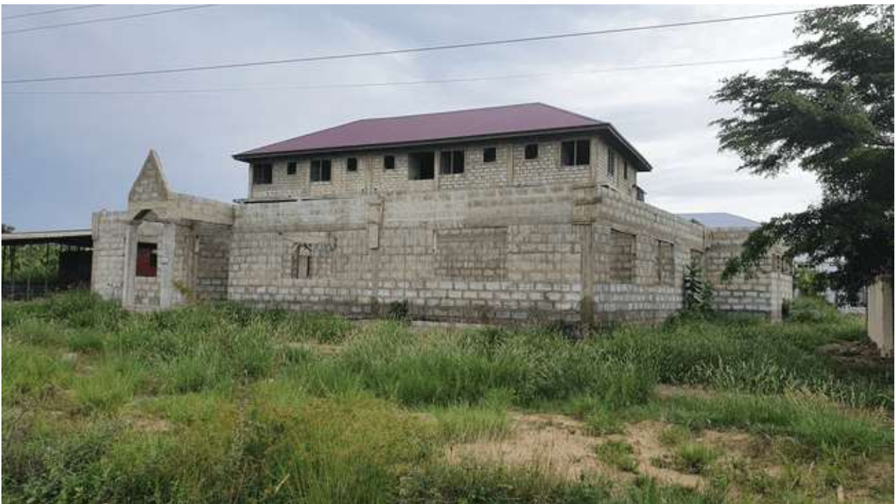
Construction of Community Library at Community 14
