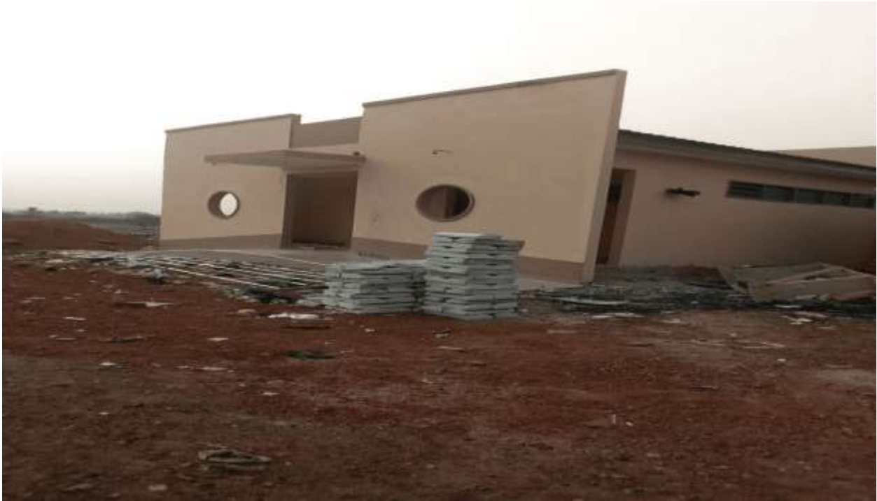
Construction of 10-Seater WC at Klagon – Ayegbekope
