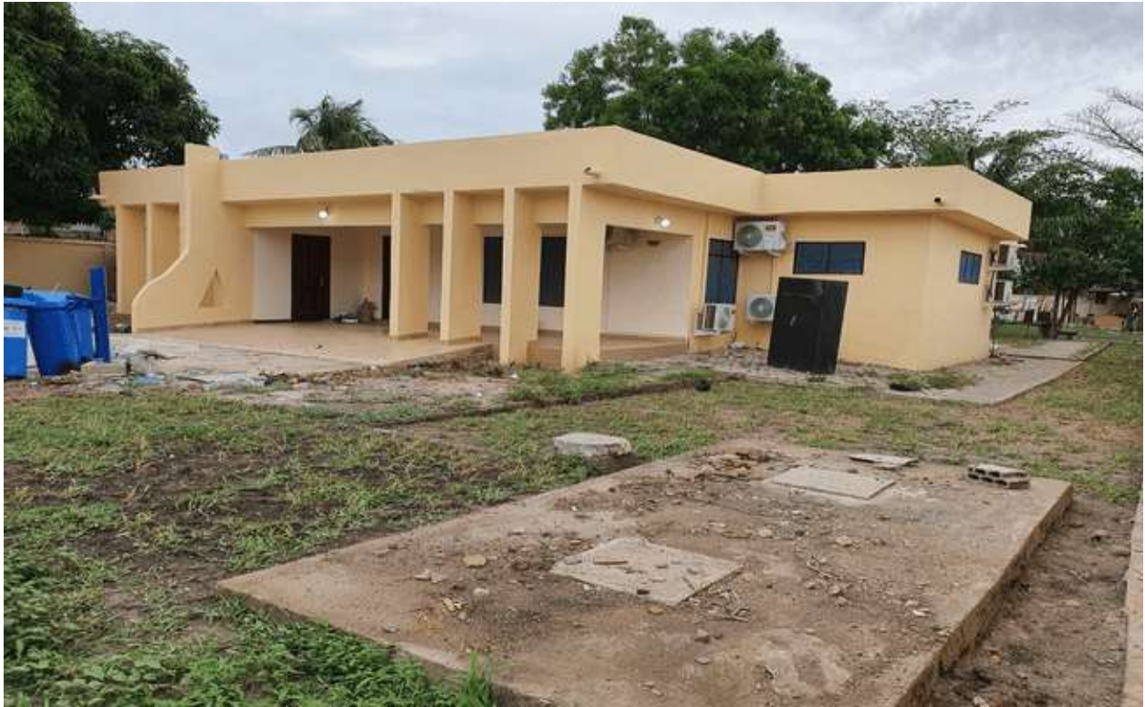
Renovation of Out House for Office at Baastonaa TWMA Main Office
