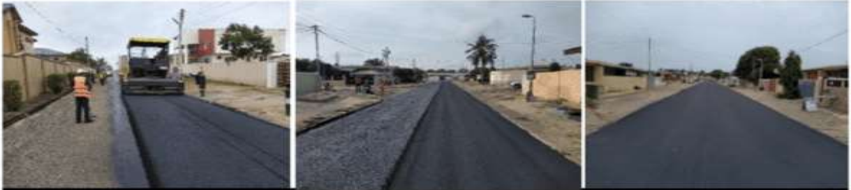
Asphalt works at Sakumono 2 nd Chapel Square link
