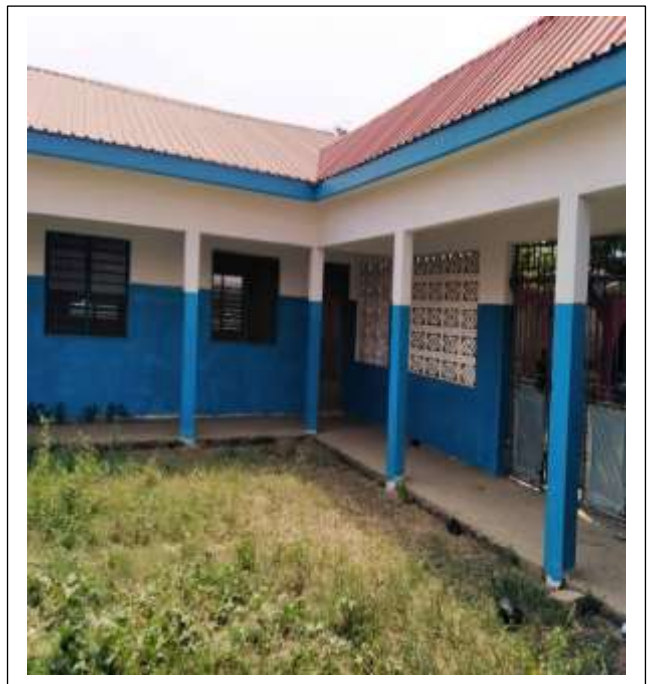
Plate 1: Construction of 6-Unit Classroom Block for Manhean Presby KG School
