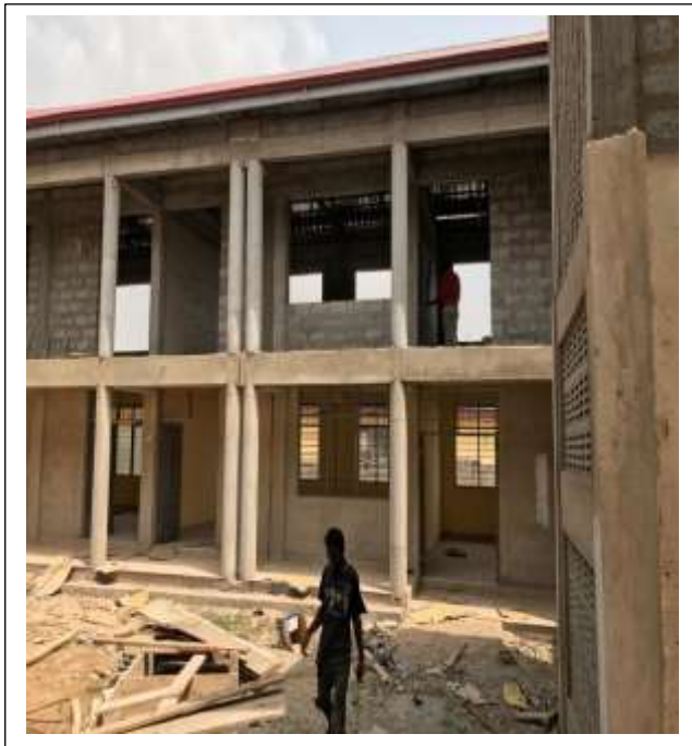
Plate 1: Construction of 12-Unit Classroom Block for Manhean Presby School
