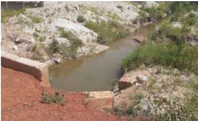
Extended Dredging Works at Metro Mass –Rahma Town
