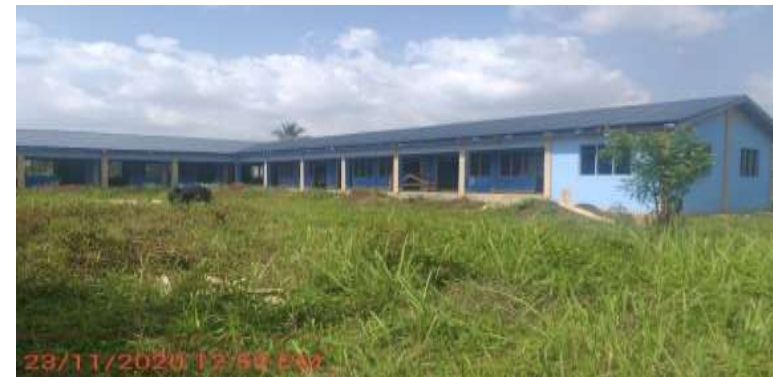
construction of 1 no 6-unit classroom block high technical asutsuare
