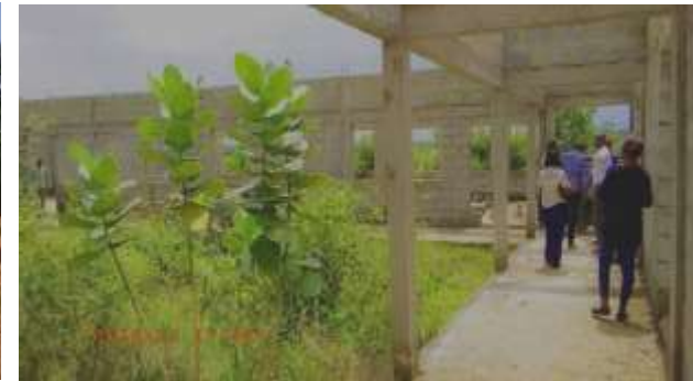
Construction of 1 No. 12-Unit Classroom Block at Osuwem
