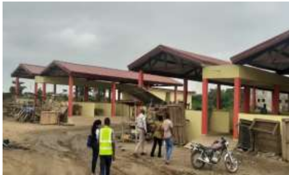
Construction of 72 No. Market Shed at Asutsuare
