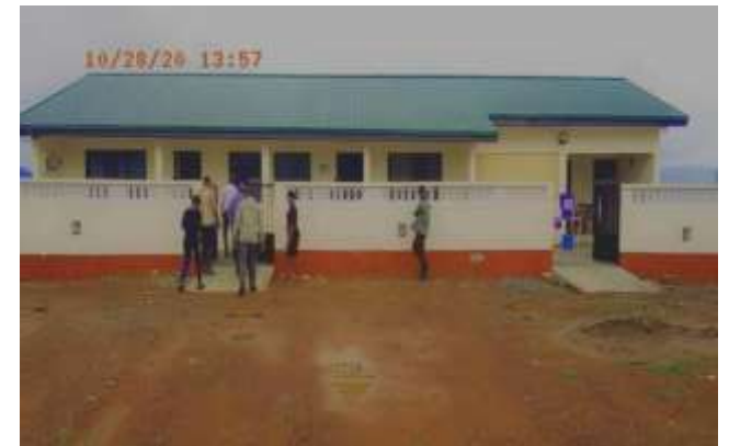
Construction of Health Centre at Doryumu
