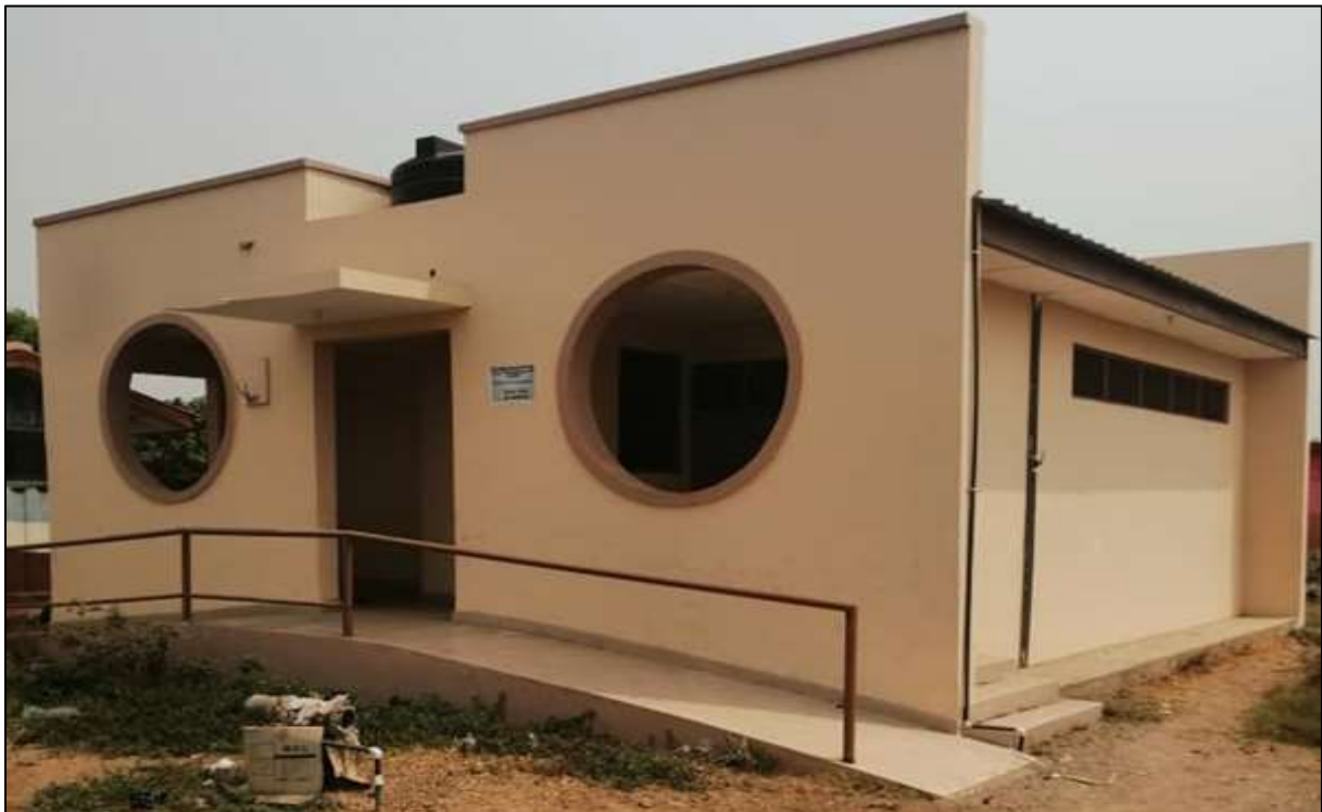
Plate 2.2: Newly Constructed Public Toilet at Afienva under the IPEP
