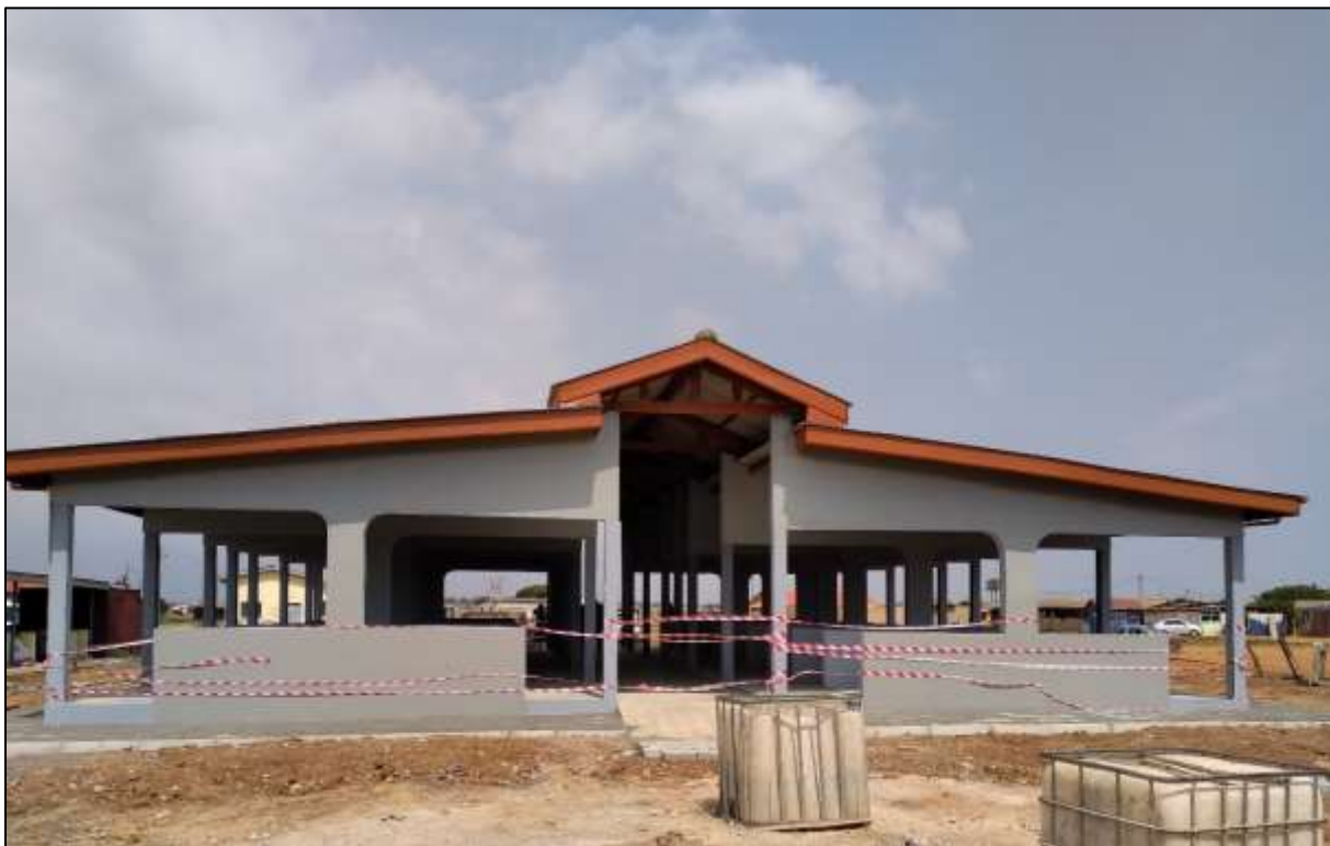
Construction of 40-Unit Market Shed at Old Ningo
