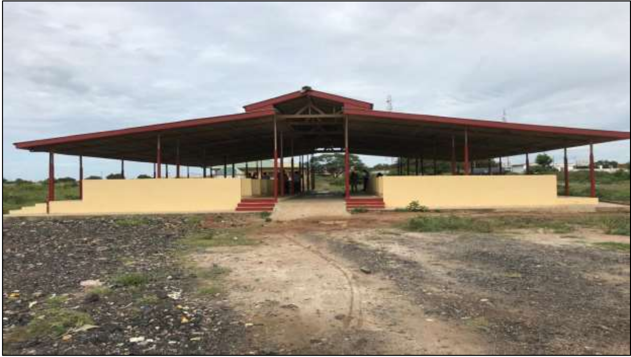
Construct 40-Unit Market sheds at Tsopoli
