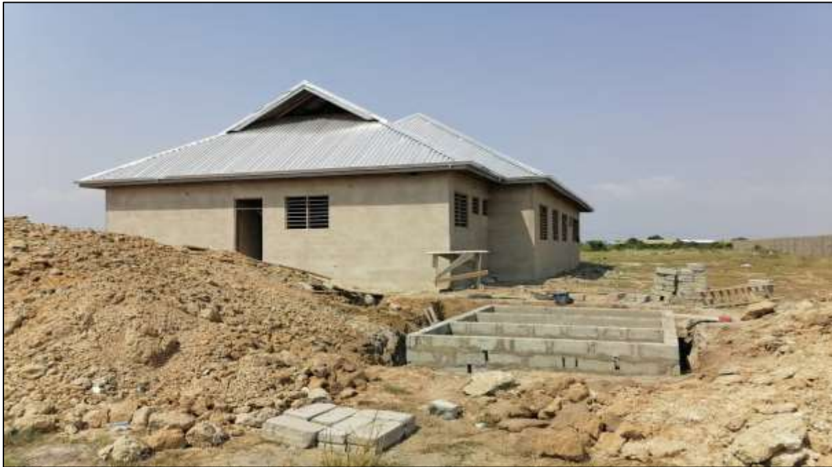
Construction of 10-Bed Maternity Ward for Old Ningo Health Center
