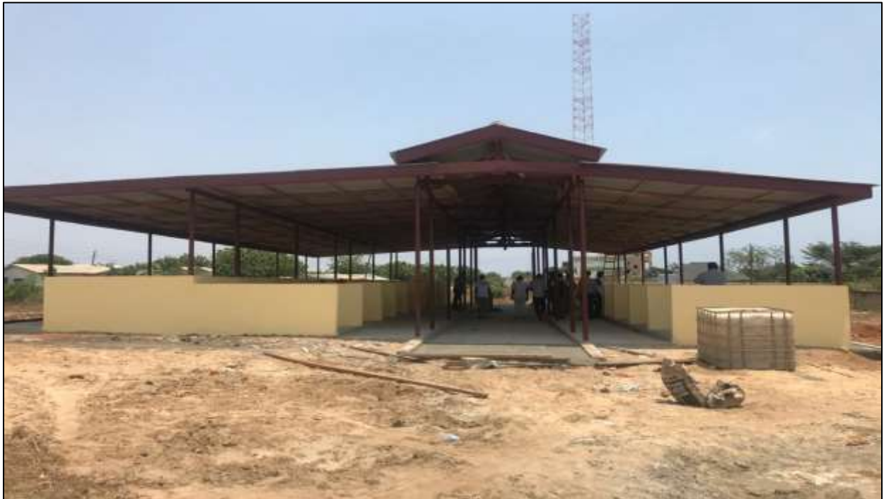
Construction of 30-Unit Market sheds at Miotso
