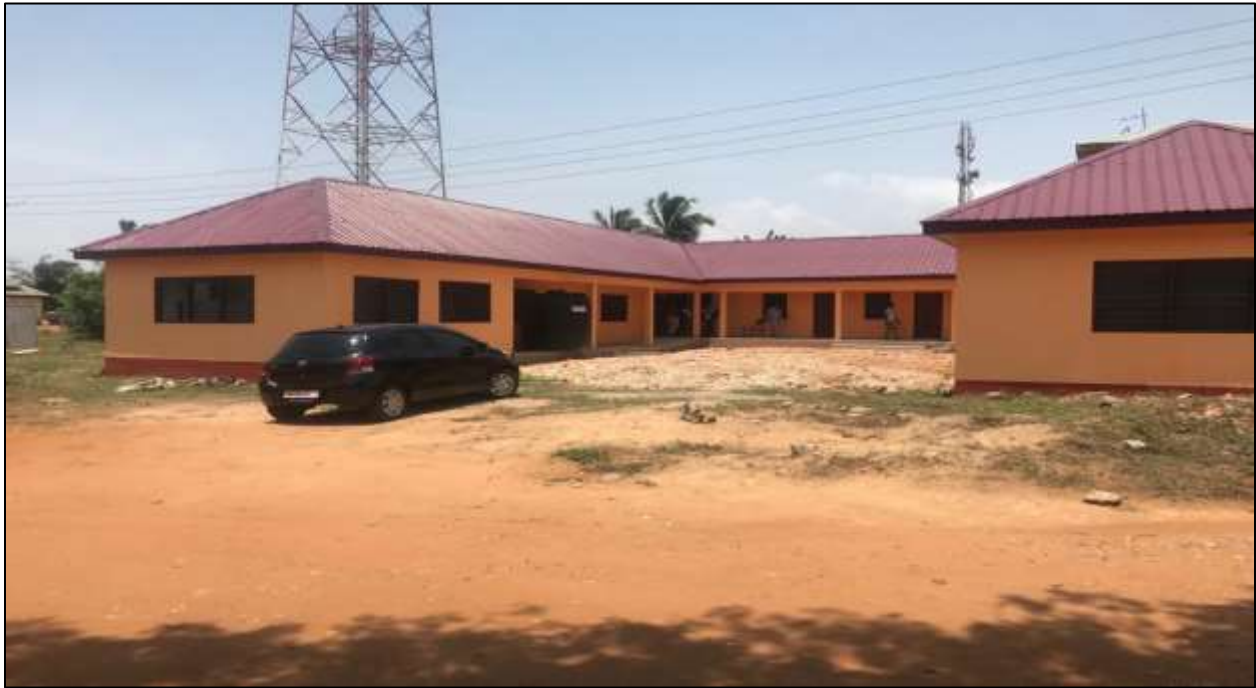
Rehabilitation of KG Block into Departmental Office Block at Prampram
