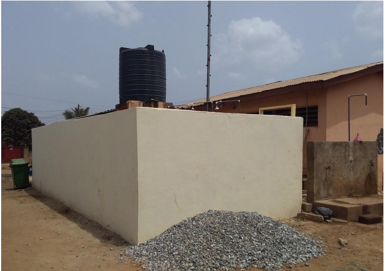
Construction of 1 No. 6 Unit Urinal at Ofankor Market
