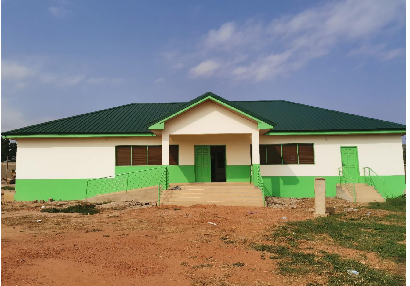
Construction of 1 No. CHPS Compound for Atiwoto Community
