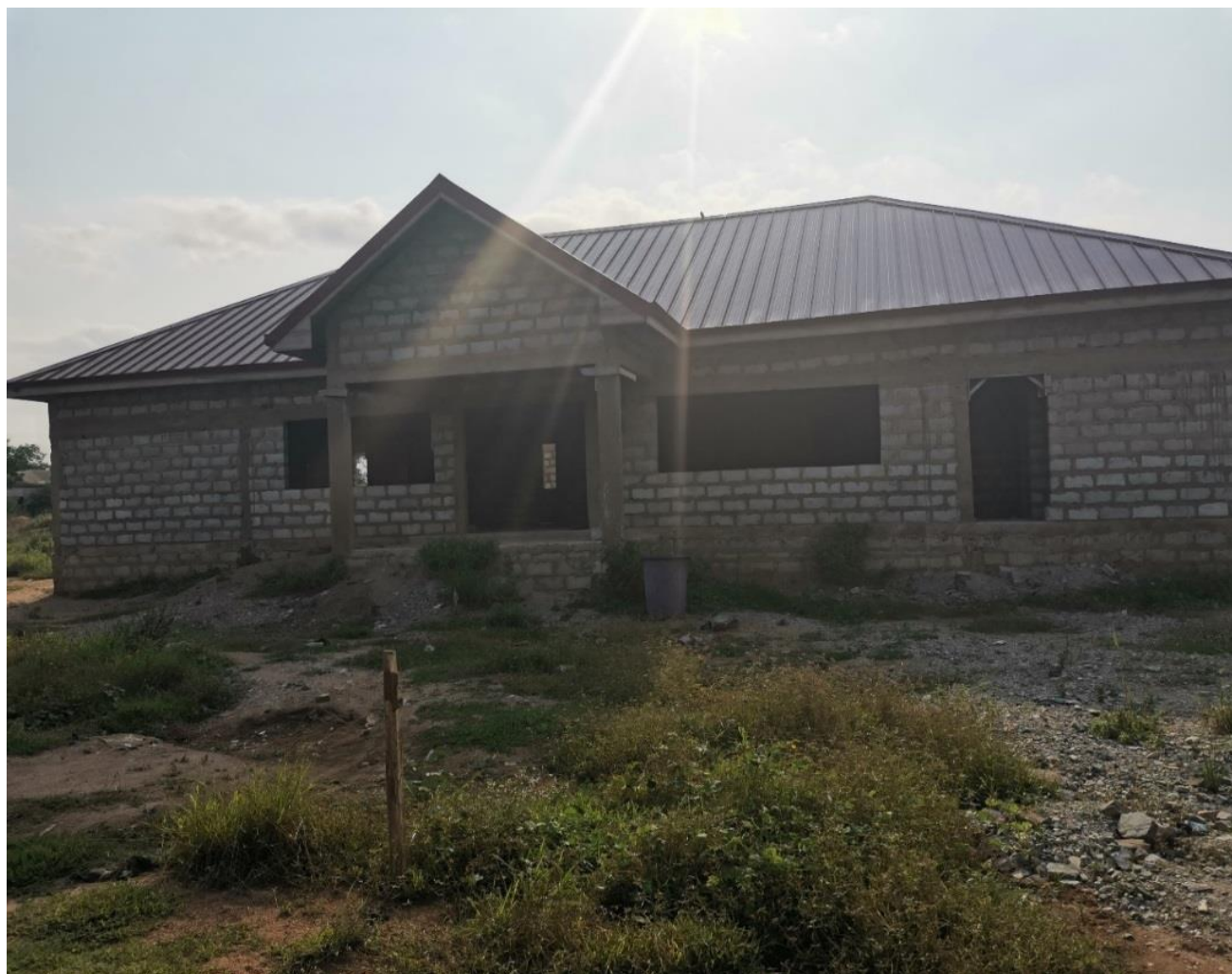
Construction of 1 No. CHPS compound for Afiaman Community
