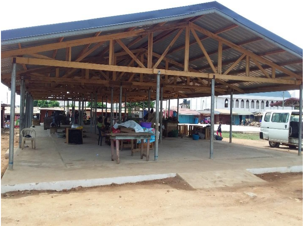
Construction of 1 No. Market Shed at Ofankor market
