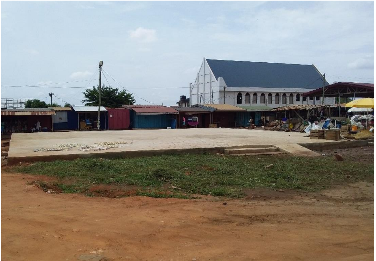
Construction of 1 No. Concrete Platform for Bulk Breakers at Ofankor Market
