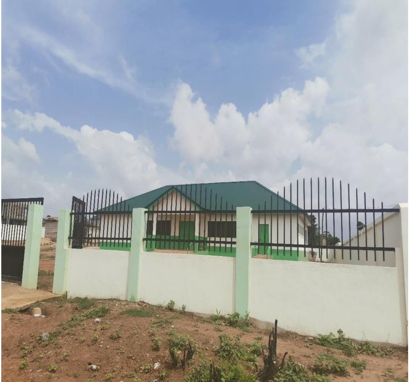
Construction of fence wall around the Atiwato CHPS Compound
