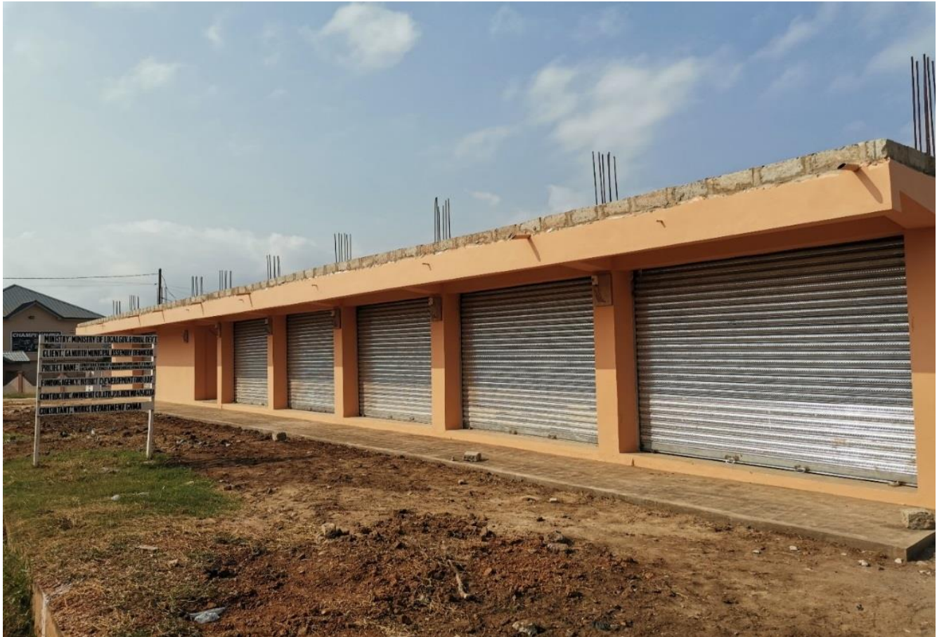
Construction of 5 unit lockable stores and warehouse at Ofankor Market
