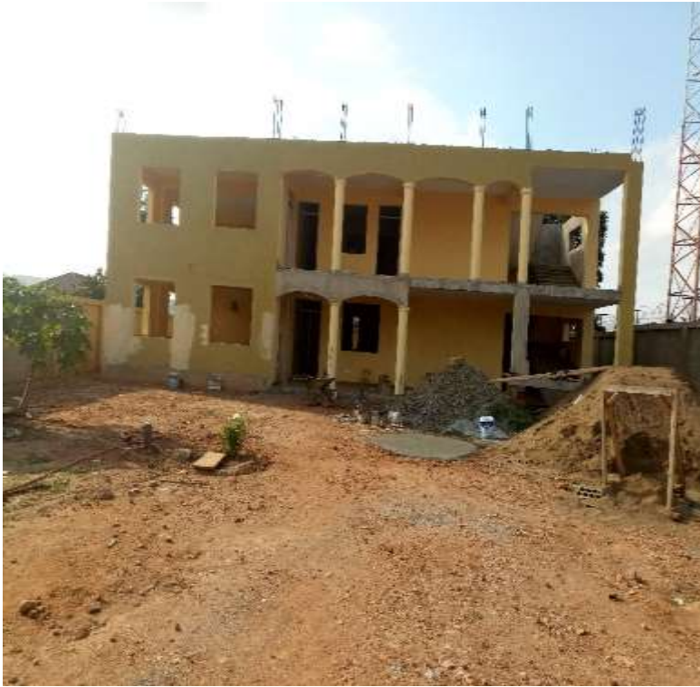
Construction of Fire Service Station at Anyaa Market
