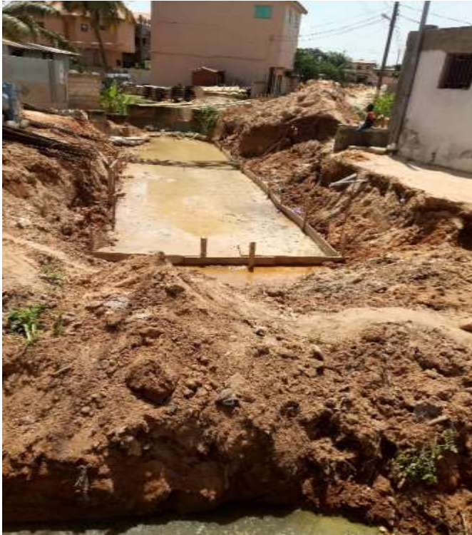
Construction of 3m× 2m Single Culvert at Sowutuom-Mambo
