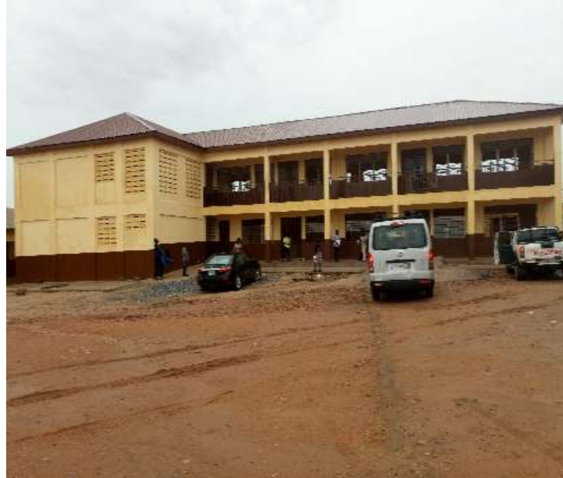
Construction of educational facility at Anyaa M/A
