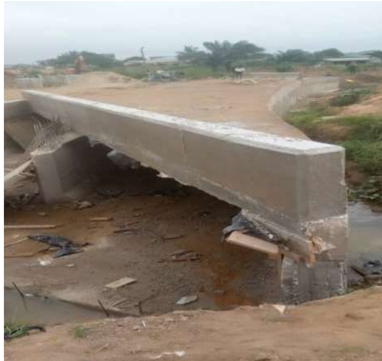
Construction of 3m× 2m Double Culvert at Olebu
