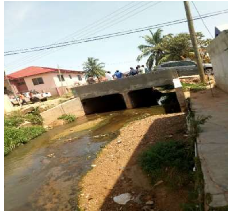
Construction of 3m× 3.2m Double Culvert at Race Course
