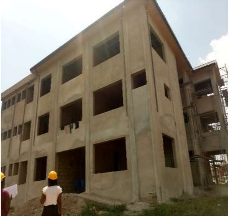
Construction of 1No. 3 Storey Clinic at Abase
