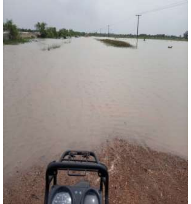
Inaccessible road to Sonkope during heavy down pours.
