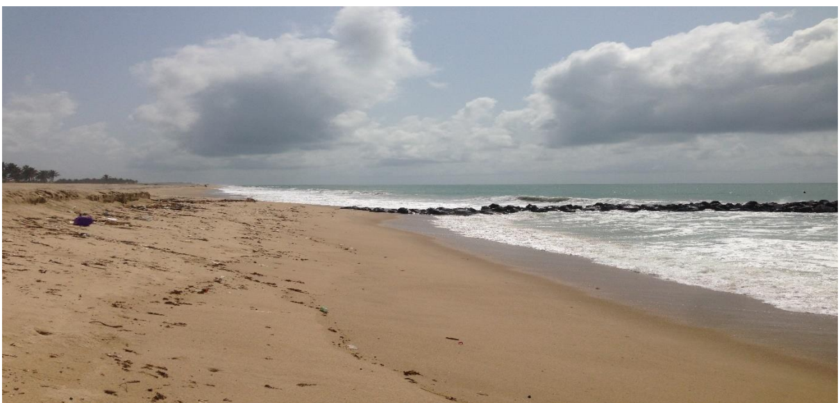
Figure 5: Reclaimed coastline after the Emergency Coastal Protection Works-June, 2015
