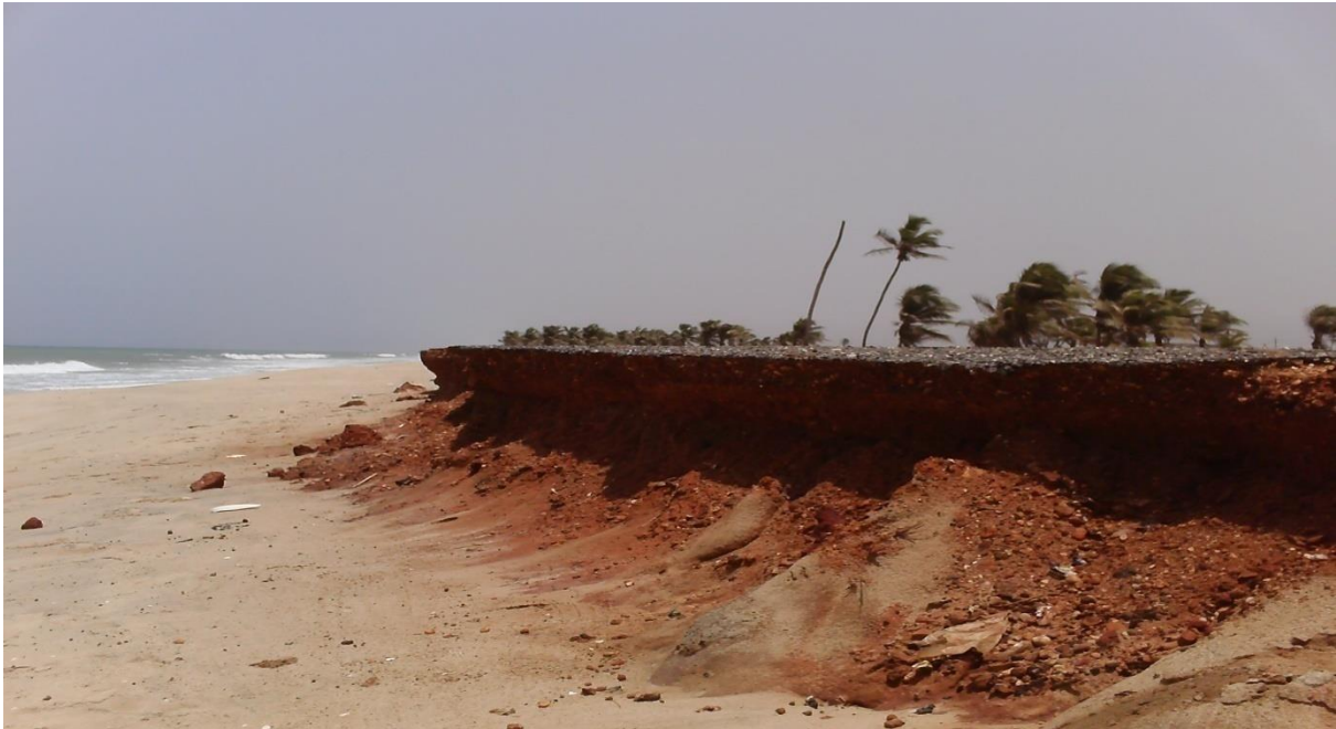
Figure 4: Devastated Ada-Foah- Otokpe thoroughfare by tidal waves
