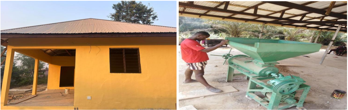
FIGURE 43: OFFICE FOR PALM OIL PROCESSING FACILITY AND EXPELLER FOR WOMEN’S GROUP AT OKAIKROM.
