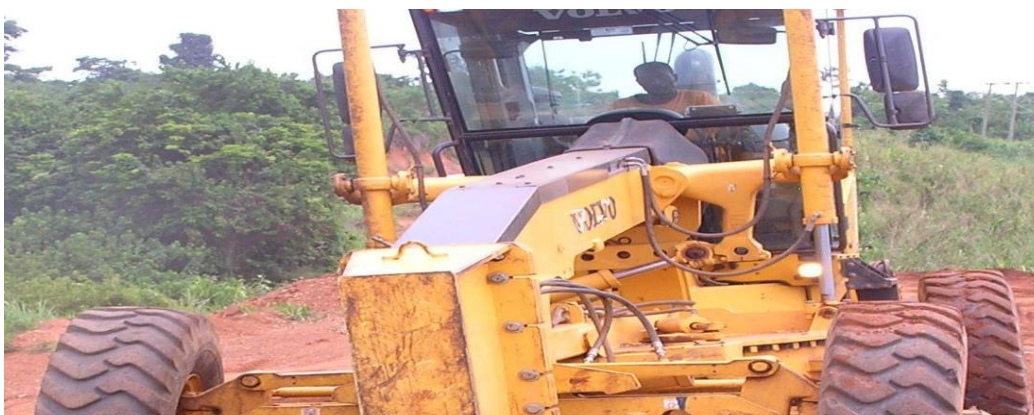
Plate 1.4: Reshaping on one of the deplorable roads in the Municipality
