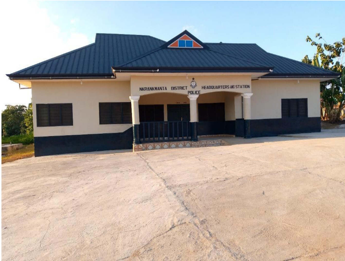
The newly commissioned District police headquarters in Nkrankwanta
