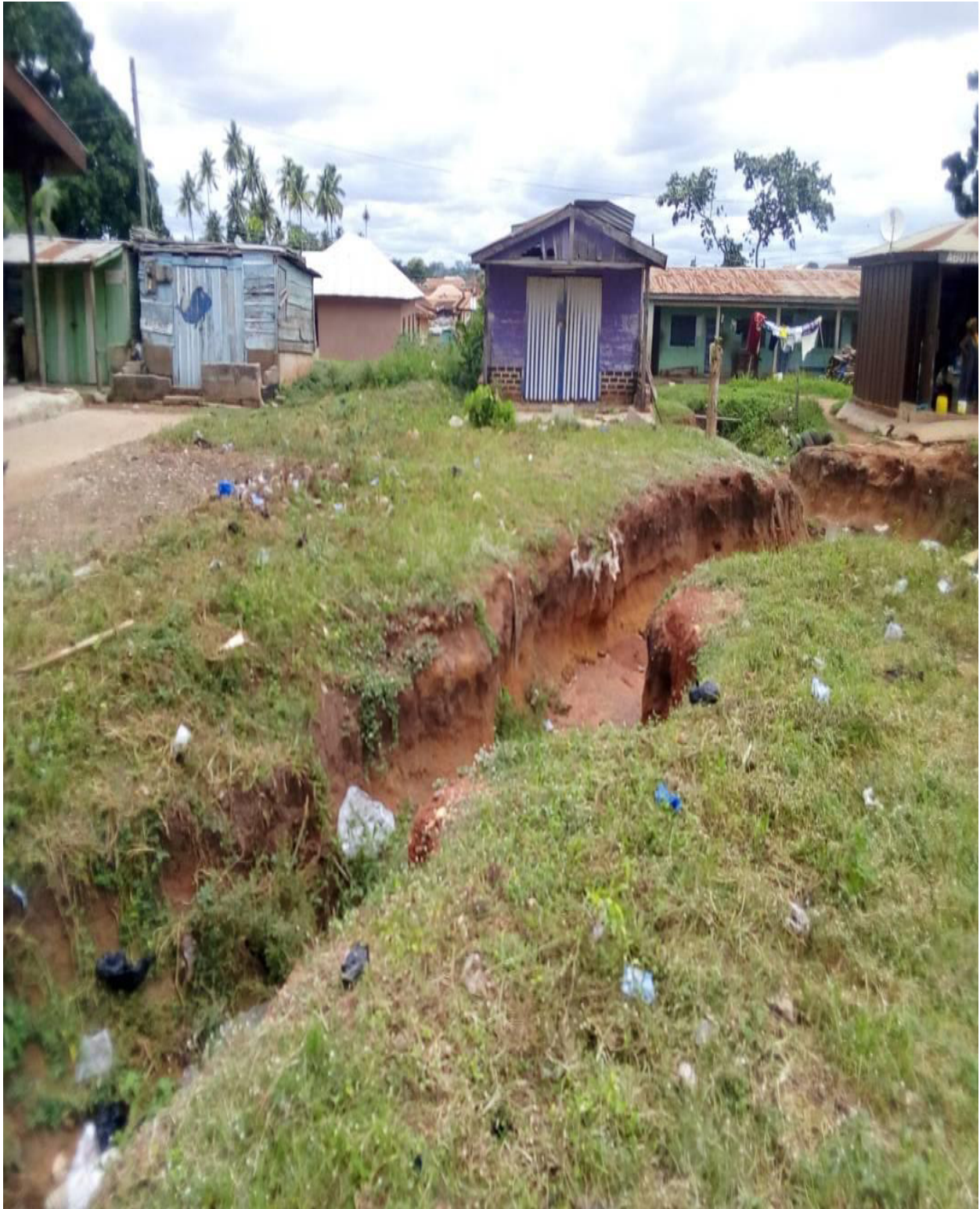
Picture 3.3: Erosion at the Jinijini market causing a large opening (drain)
