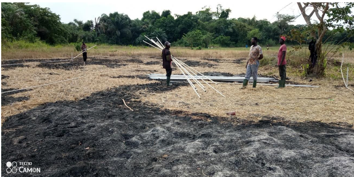
Assembling of Irrigation pipes at Asuano
