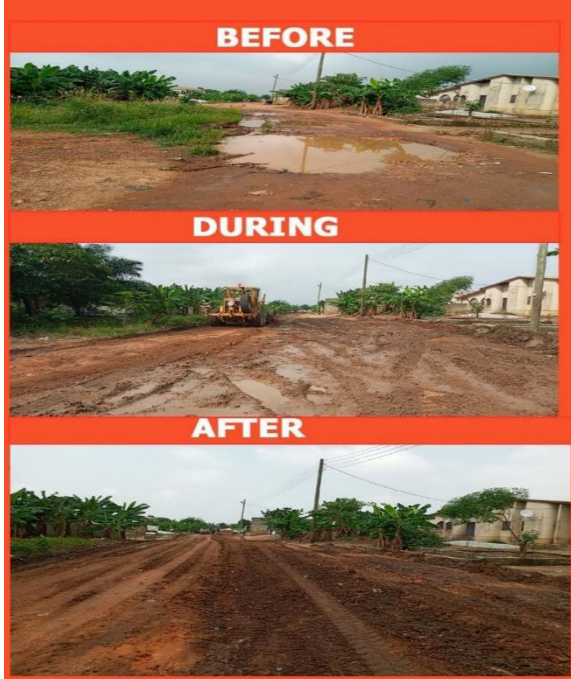
Figure 2.9 C: Grading Works at Abouhia
