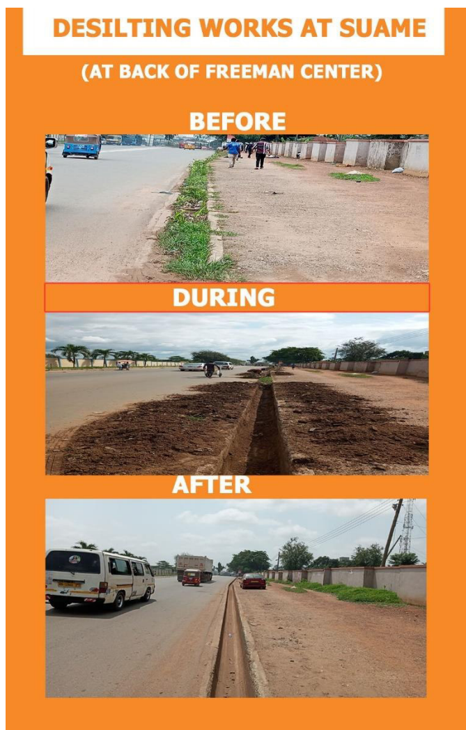
Figure 2.7(A) Desilting of choked drains
