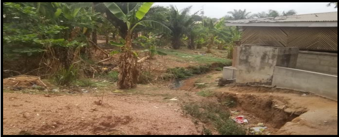
Plate 1.7: Effects of Erosion
