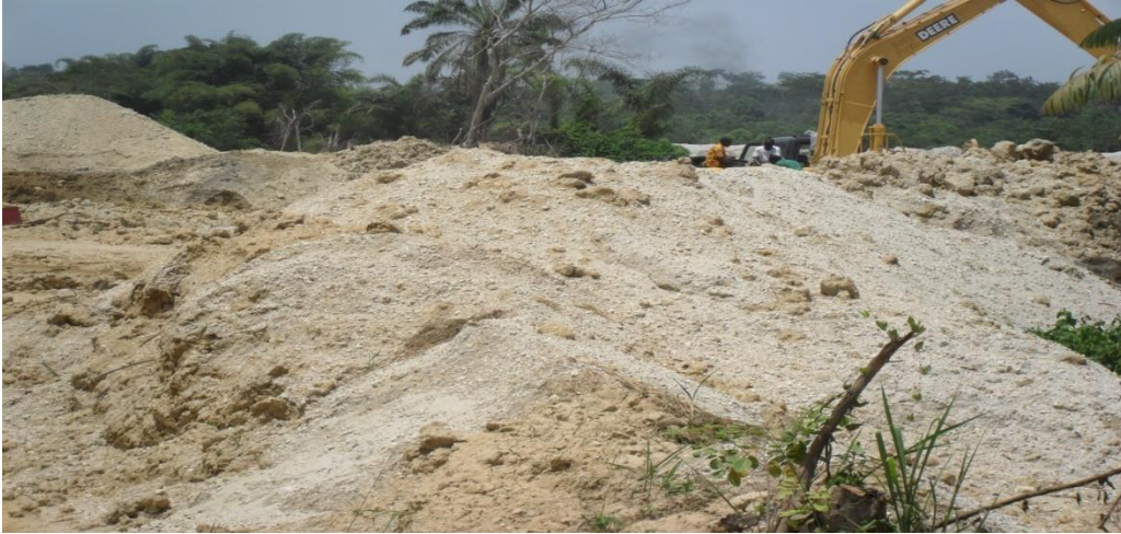
Plate 1.4: Sand Dumped for reclamation
