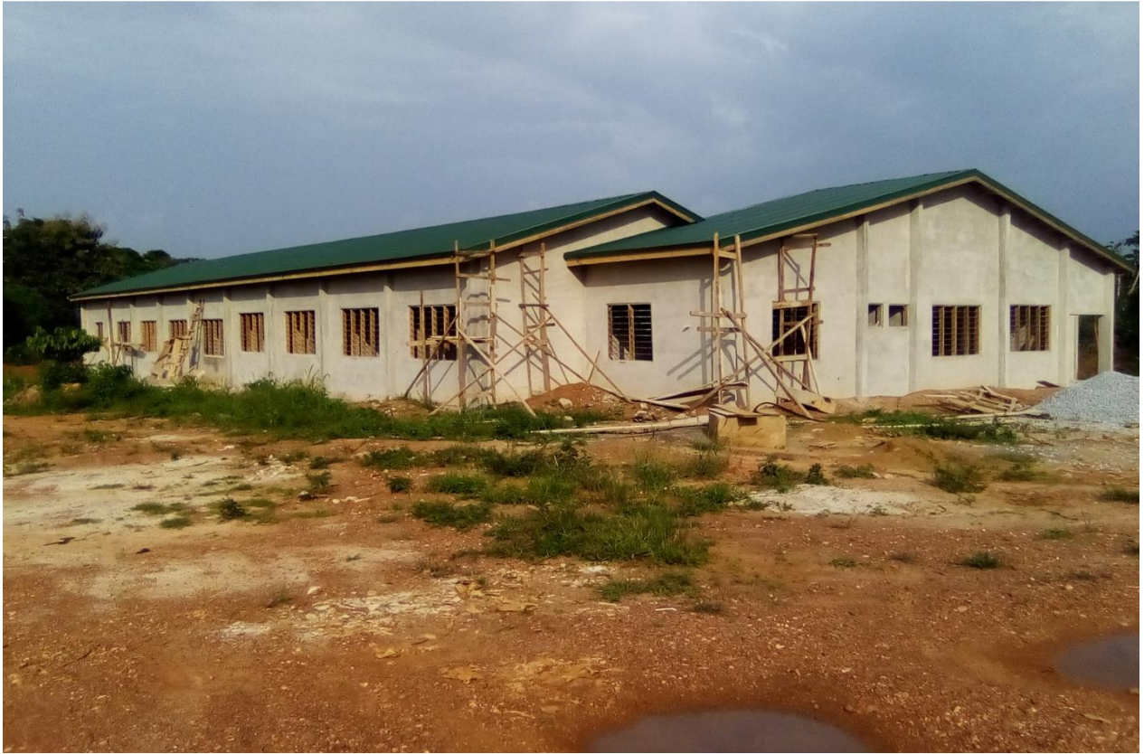
Construction of 1No.12-Unit Dormitory at Dadiesoaba Nursing Training (Middle Belt Authority)
