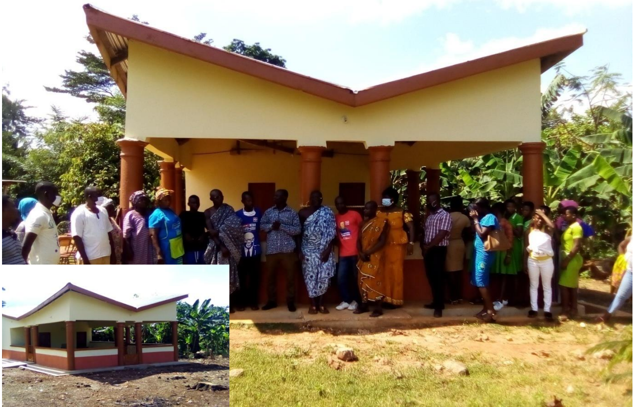
Construction of 2 No. Weighing Centres at Ayago and
