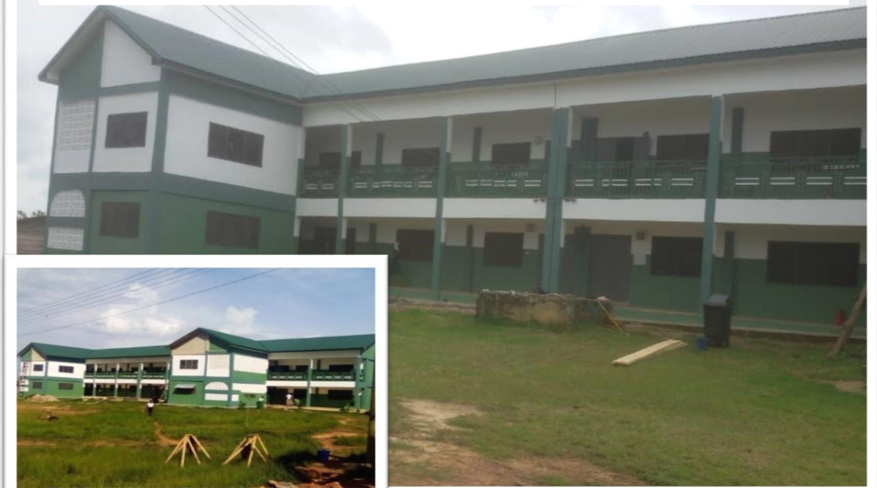
Construction of 1No.12-Unit Classroom at Dadiesoaba Nursing Training (GETFund)
