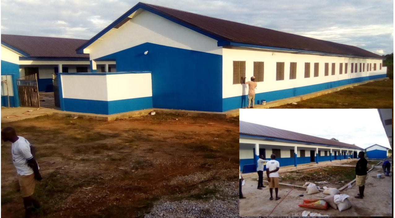
Construction of 1No.12-Unit Dormitory for Boys at Acherensua SHS (GETFund)
