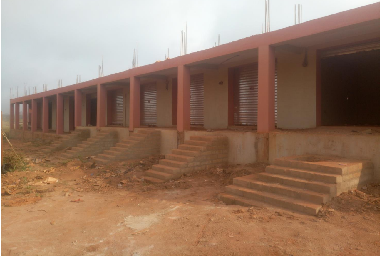
Construction of 1No. 10-Unit Lockable Market Stores at Hwidiem (DPAT Project)
