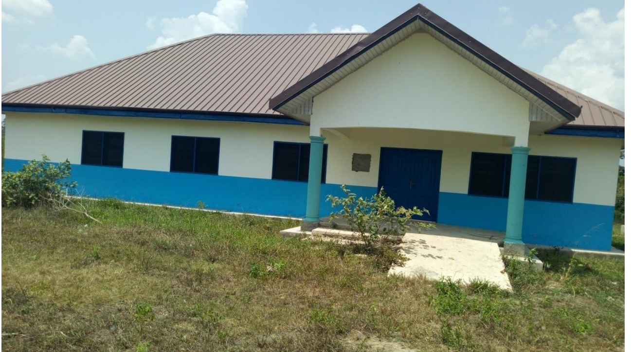
Construction of 1No. Rural Clinic with Mechanized Borehole at Woramumuso (SIF/IGF)
