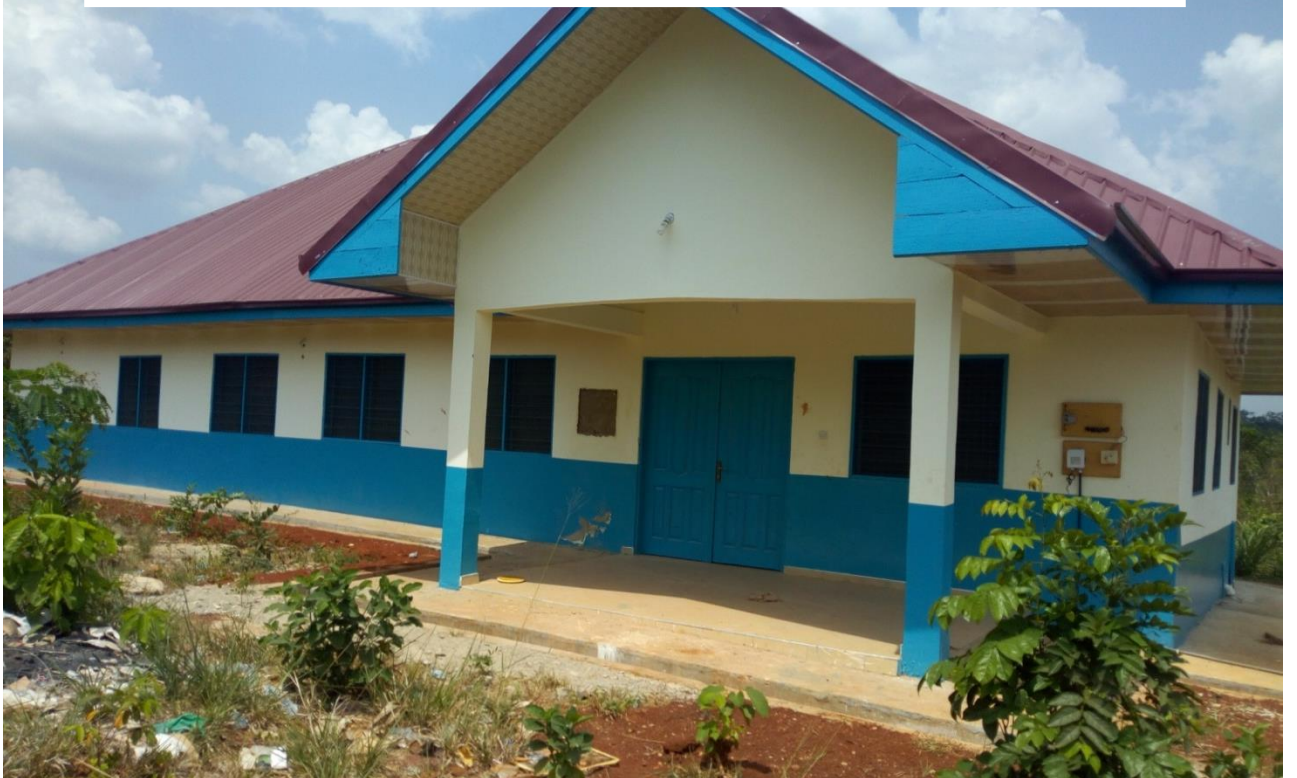
Construction of 1No. Rural Clinic with Mechanized Borehole at Mehame (SIF/IGF)
