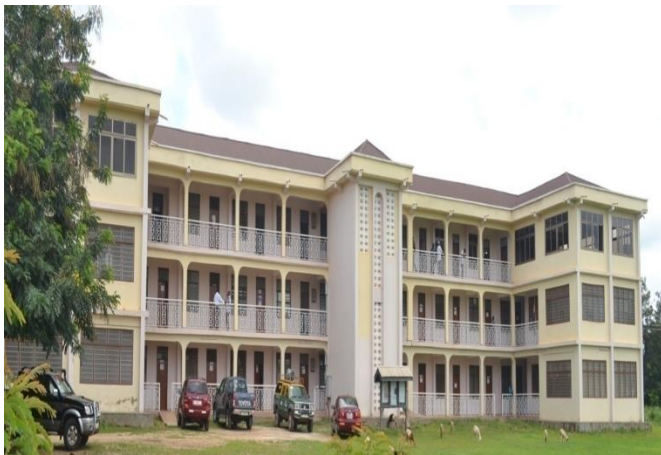
Main Administration Block Housing Finance, Works, Physical Planning and Others
