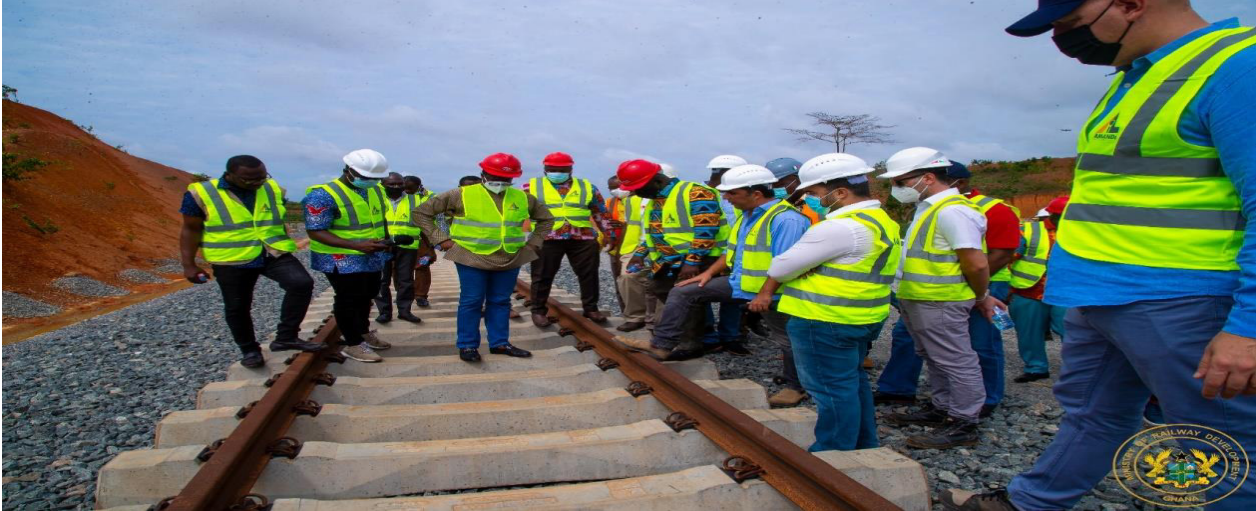
Figure 2.28: On-going Construction of the Kojokrom-Manso Section of the Western Line
