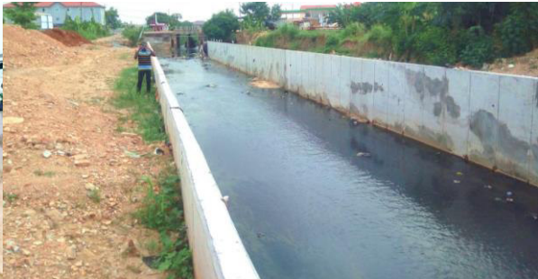
Figure 2.36: Haatso Drainage Project
