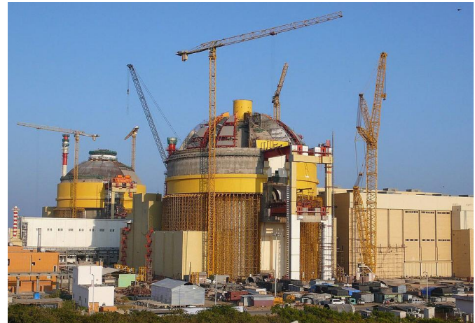
Figure 3.12: Construction of a nuclear Plant
